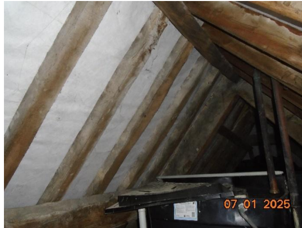
Photo 36: Internal of void 1.
