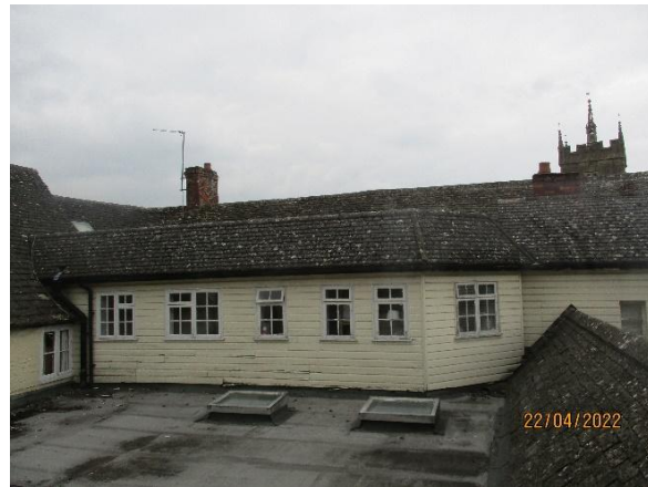
Photo 11: The upper half of the of the southernmost pitched and hipped roof in the north with concrete roof tiles.
