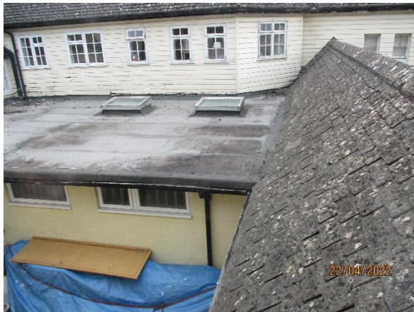
Photo 10: Flat roof extension south of the northern roofs.
