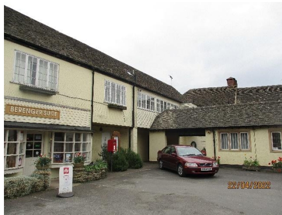
Photo 5: Porch area on the eastern elevation of the hotel.
