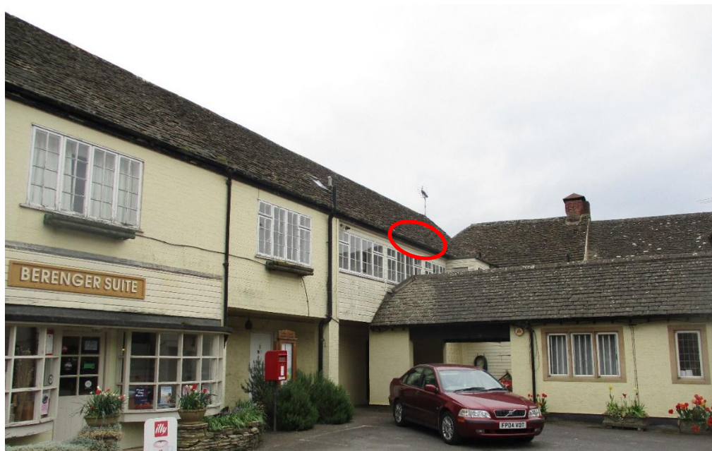
Figure 1: Location of common pipistrelle emergence.
