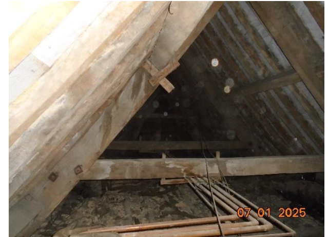
Photo 37: Internal of void 2.
