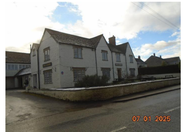
Photo 40: Front elevation of the existing hotel building from the road.
