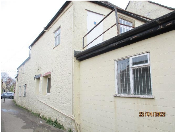
Photo 7: West elevation of the rear extension
