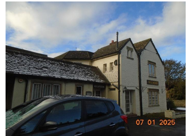
Photo 37: Existing hotel building.
