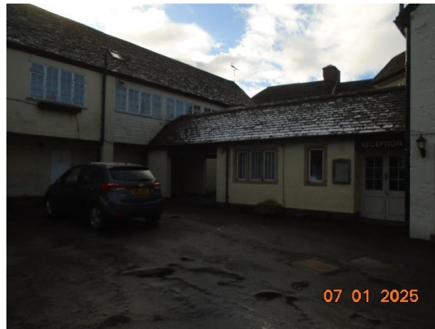
Photo 36: Front eastern elevation of the existing hotel.
