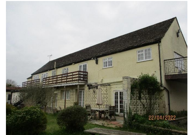
Photo 3: Rear southern elevation of the hotel.
