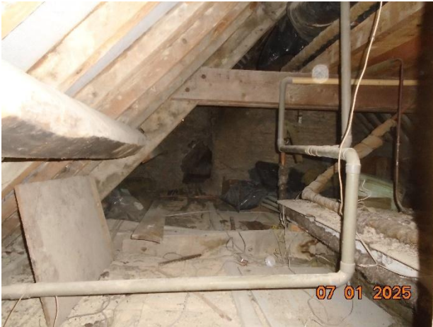
Photo 35: Internal of void 1.
