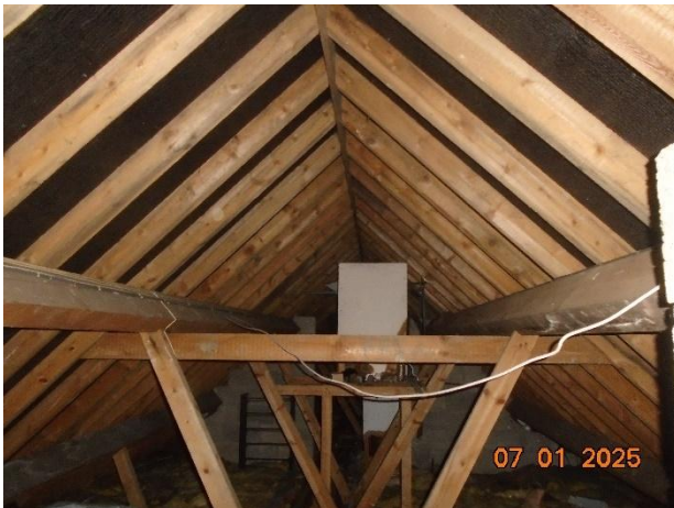
Photo 38: Internal of void 5.
