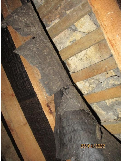
Photo 31: Area of the roof of 'Void 3' where the bitumen lining turns to no lining.
