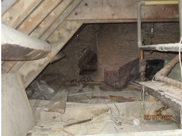
Photo 25: Internal of 'Void 1'.
