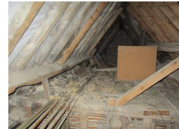
Photo 30: Internal of 'Void 2'.
