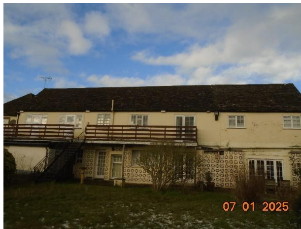
Photo 42: South elevation of the hotel to be demolished.
