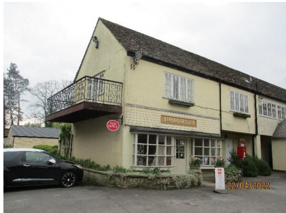
Photo 4: Side eastern gable end at the southern end of the hotel.
