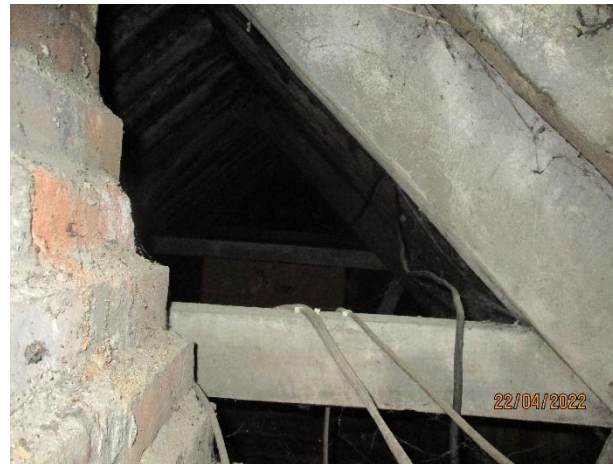
Photo 34: View of Void 4 which was inaccessible.
