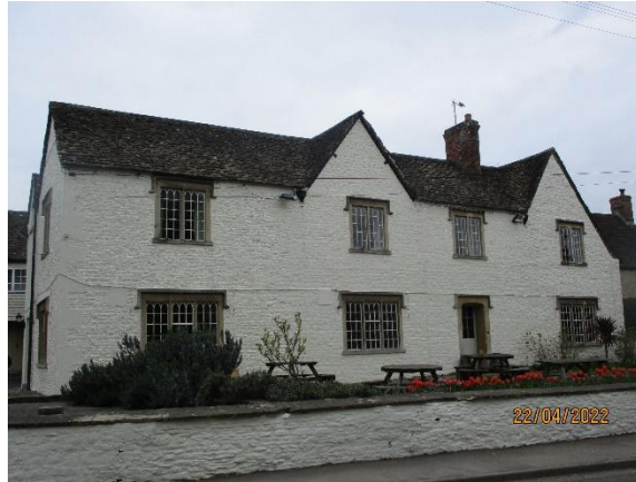
Photo 2: Front northern elevation of the hotel.
