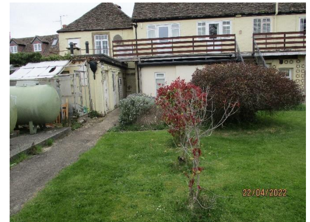
Photo 12: Rear of the hotel on the west side.
