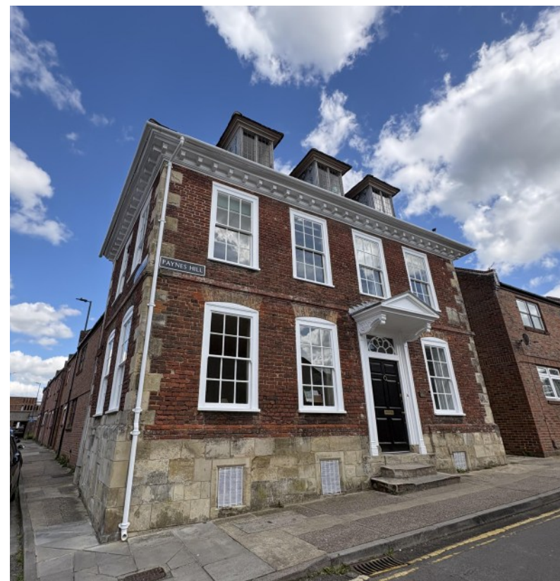
Front Façade of building
