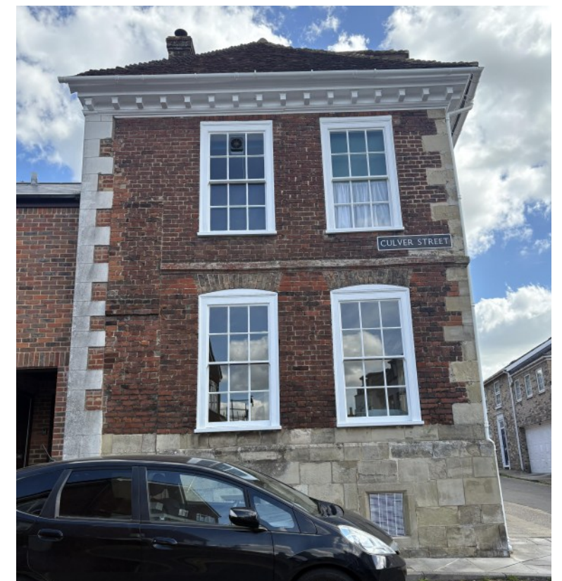
Side Façade of building
