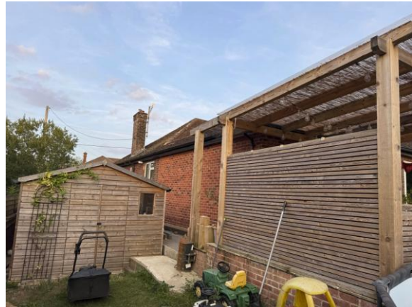
Photo 2 – View of Building 1 from the position of surveyor 2.
