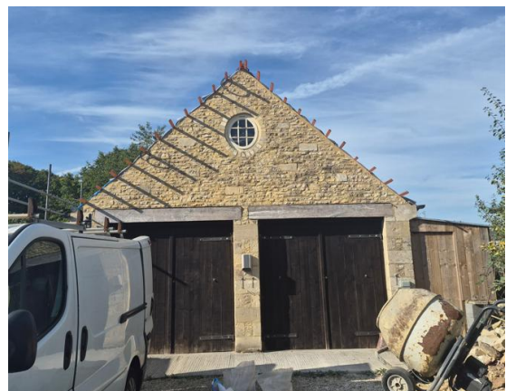
Front Façade of Existing Garage (Case Officer Site Photo)
