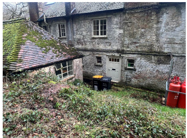
Plate 4 terrace behind Estate Office (looking SW)
