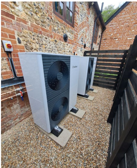
Figure 2: 2 x Vaillant Arotherm Plus, at Box Hill, Surrey (Left), Example Volta 24kW Unit (Right).
