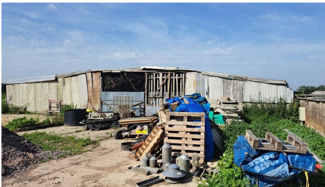
Existing building east elevation
