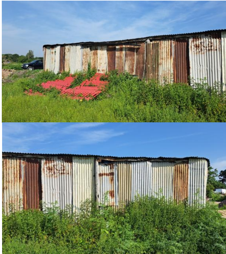
Existing building south elevation
