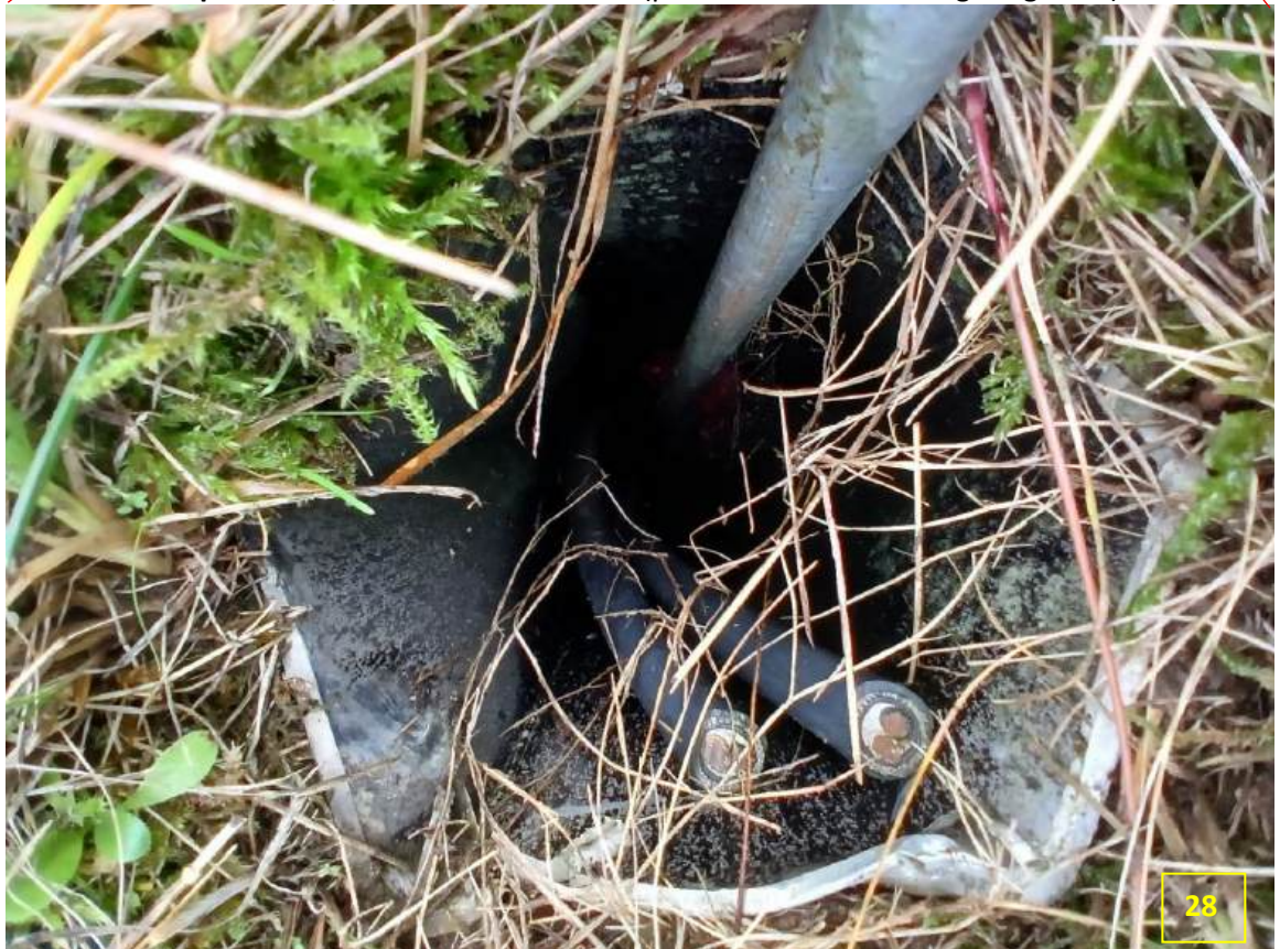
Unprotected, cut-off electric cables (possible former flood lighting mast)
