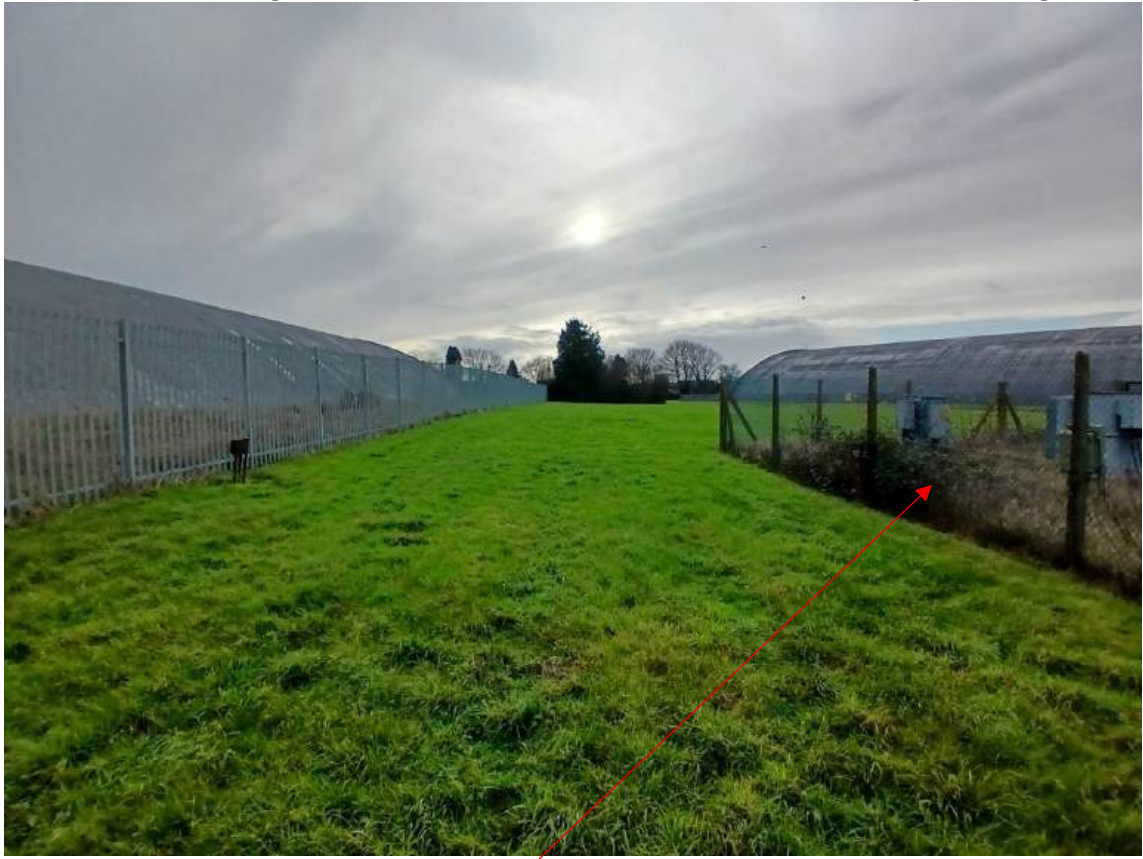
West side of hangar 19 (left) & Electric transformer/ switch station (right) (Facing S)
