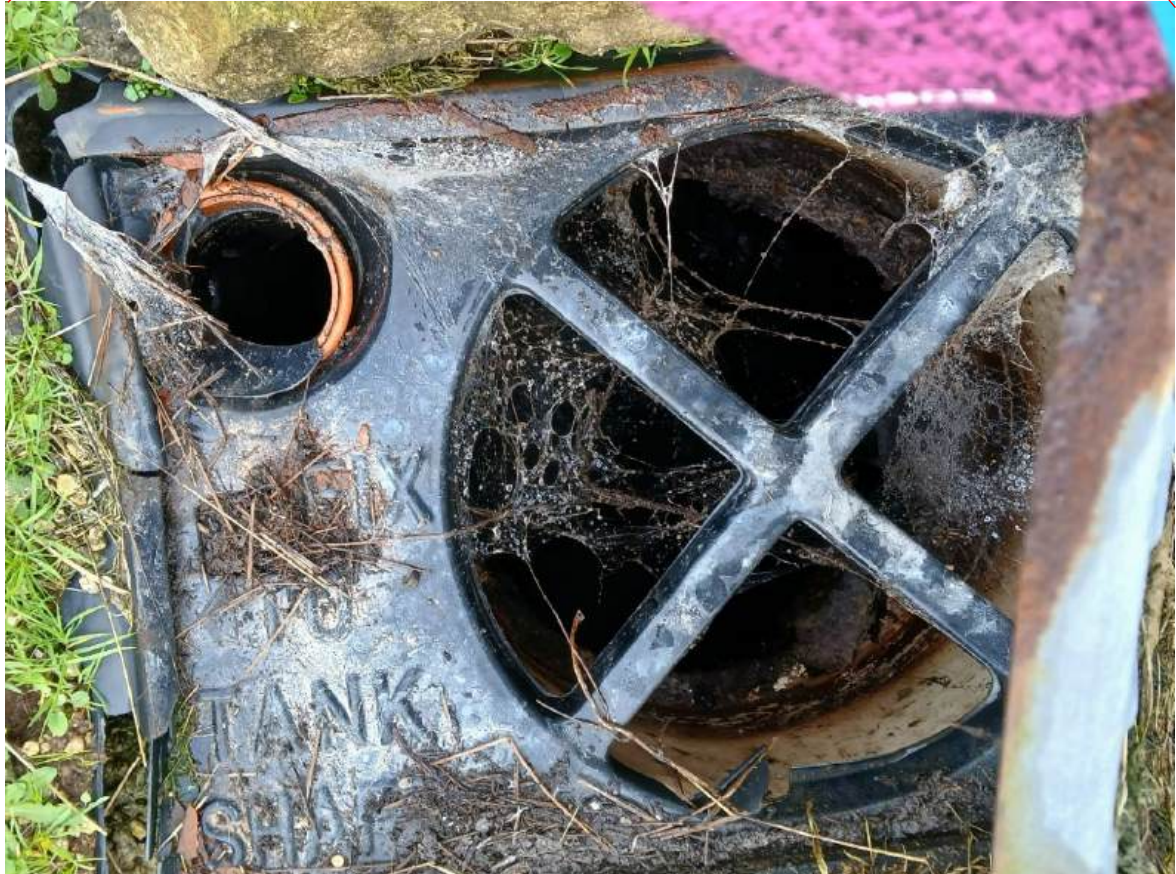
Septic tank (filled) (cover damaged)
