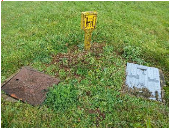
Underground fire hydrant at hangar 18
