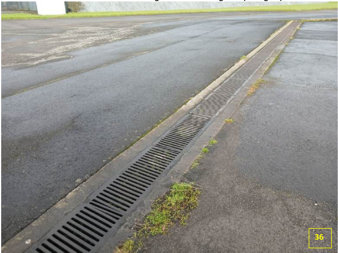
Surface water runoff drainage in front off hangar 20 (Facing NE)
