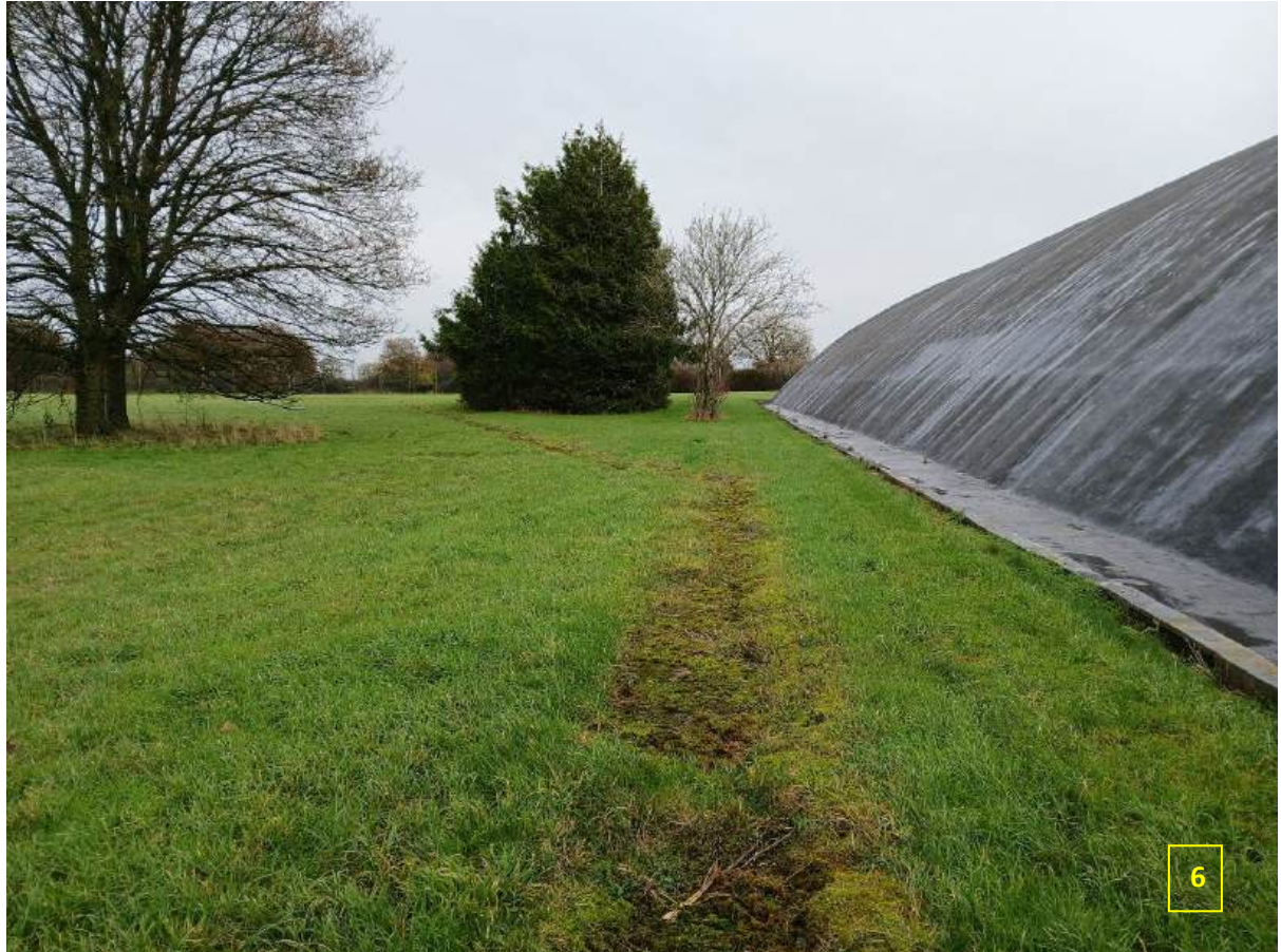
Overgrown concrete path alongside hangar 18 (Facing E)
