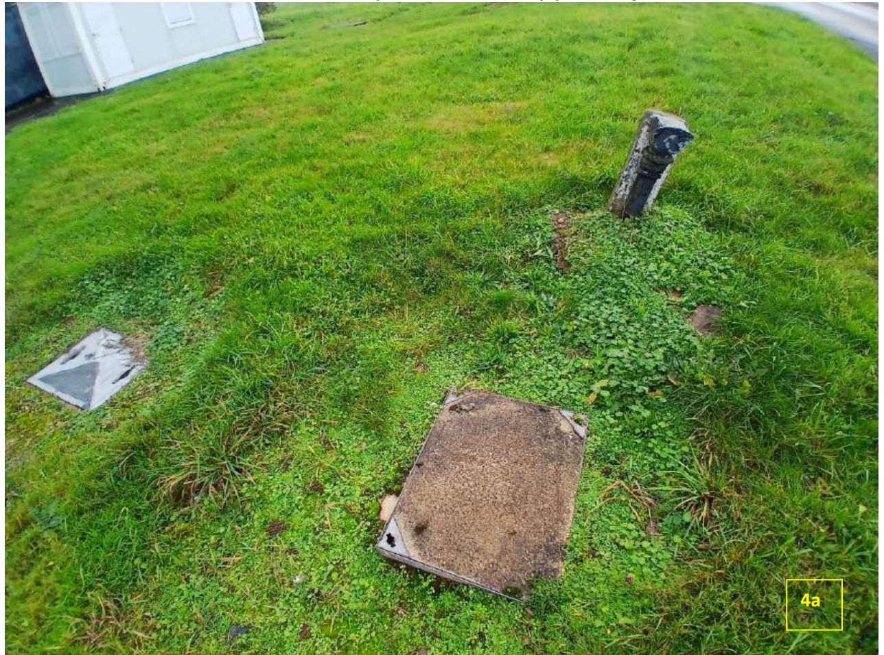
Manhole covers and possible black vent pipe (Facing NW)
