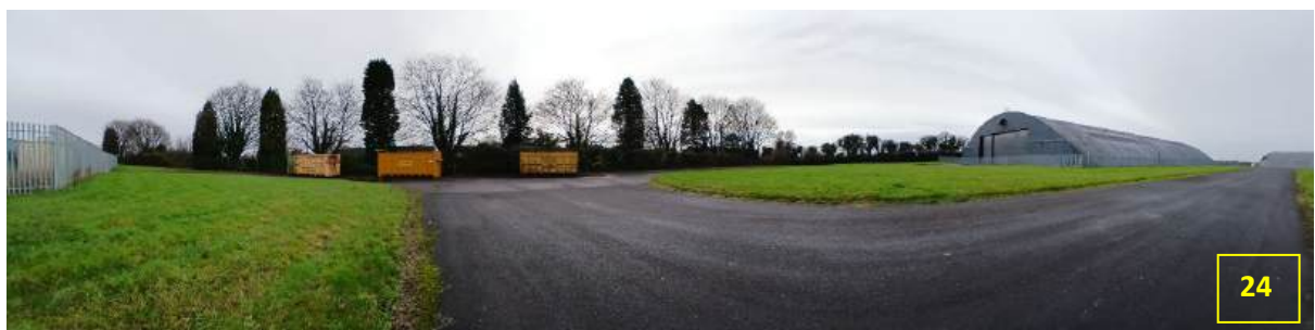
Rear of hangar 19 (left) & rear of hangar 20 (right) with access road (Facing S)
