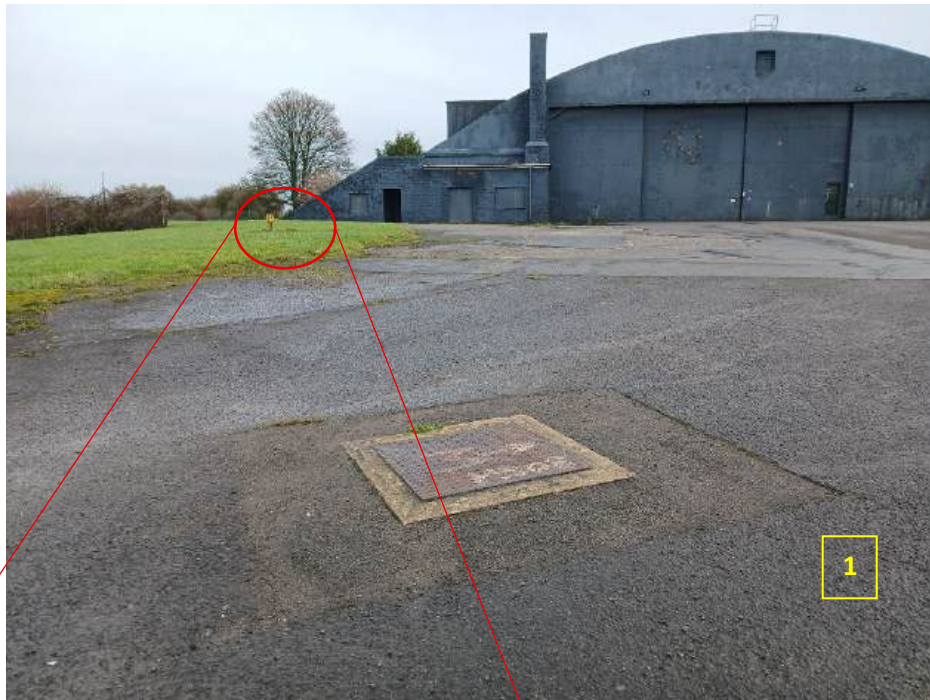
Underground fire hydrant at hangar 18
