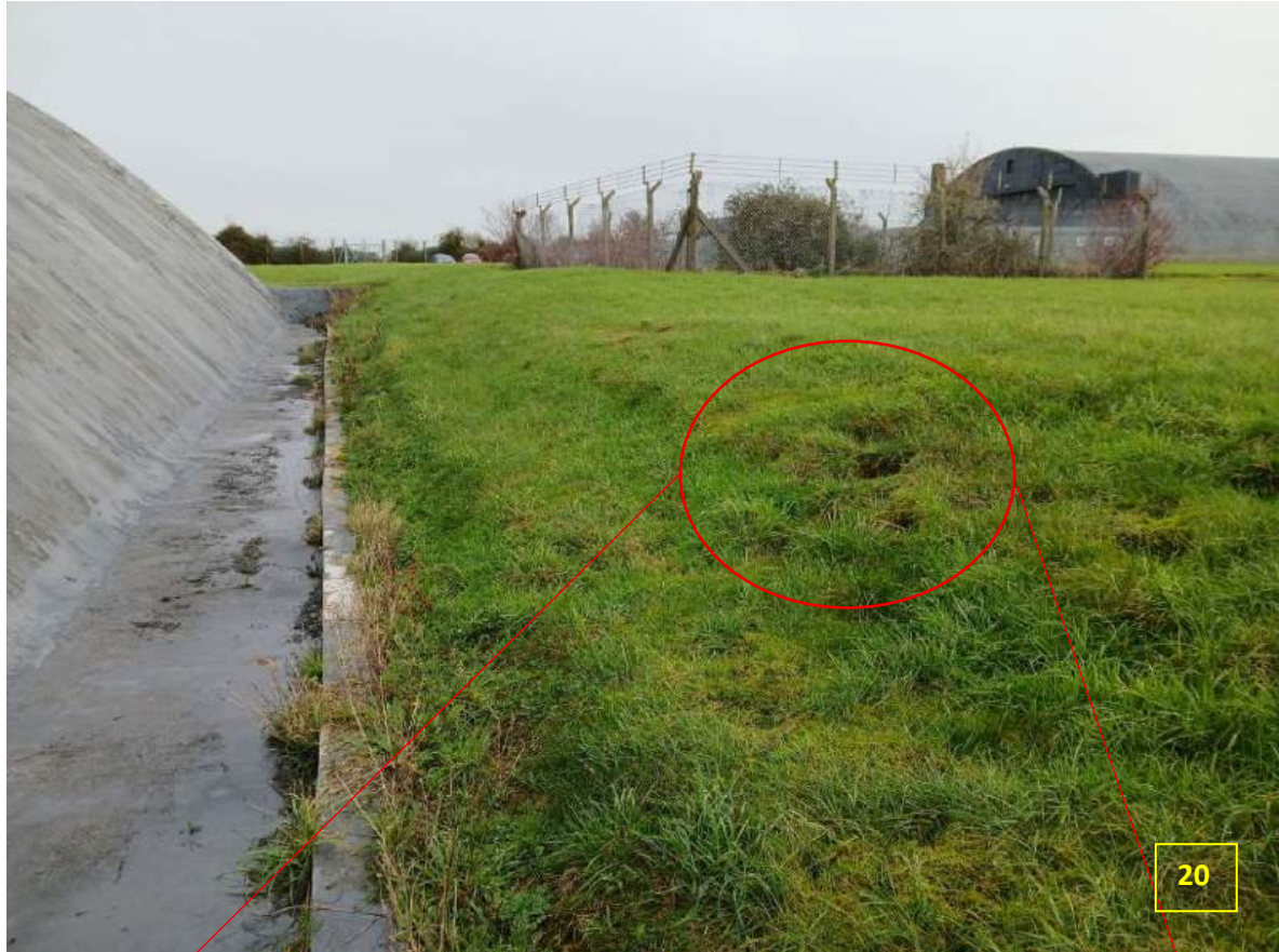
Slight embankment south of hangar 18. View towards storage basin and hangar 19
