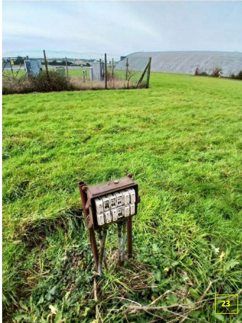
Assumed disused electric fuse board (Facing SW)
