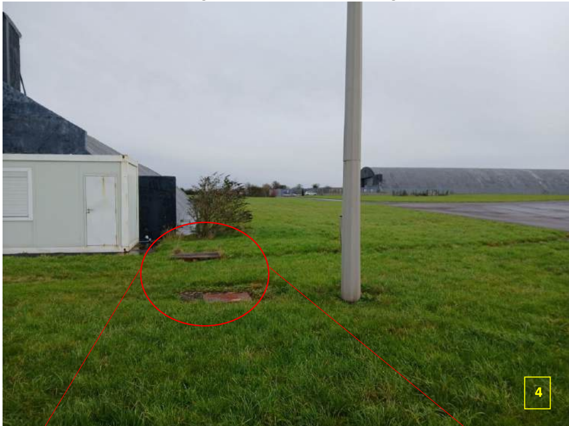
Floodlight and manhole covers (Facing E)
