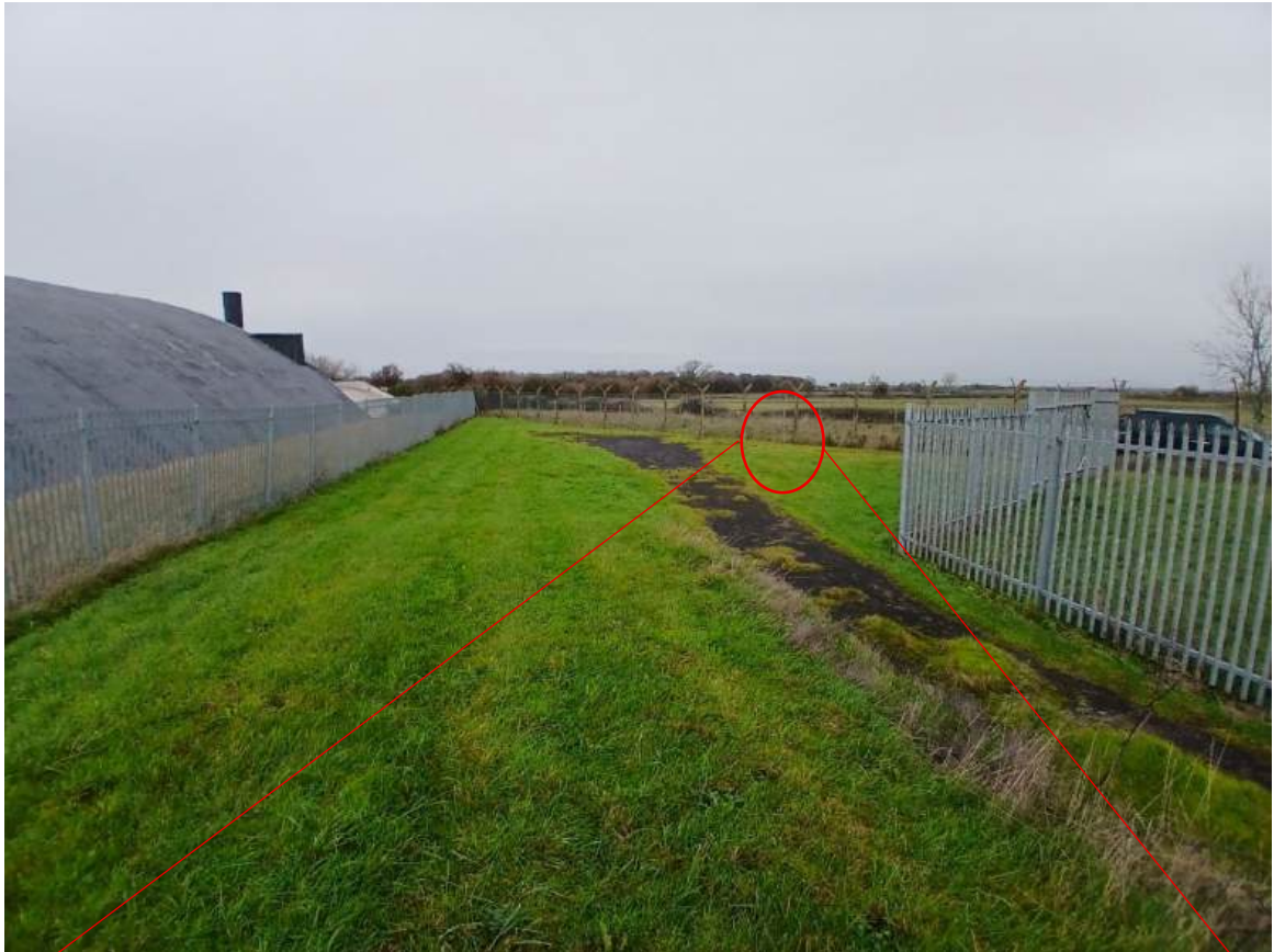
Unprotected, cut-off electric cables (possible former flood lighting mast)
