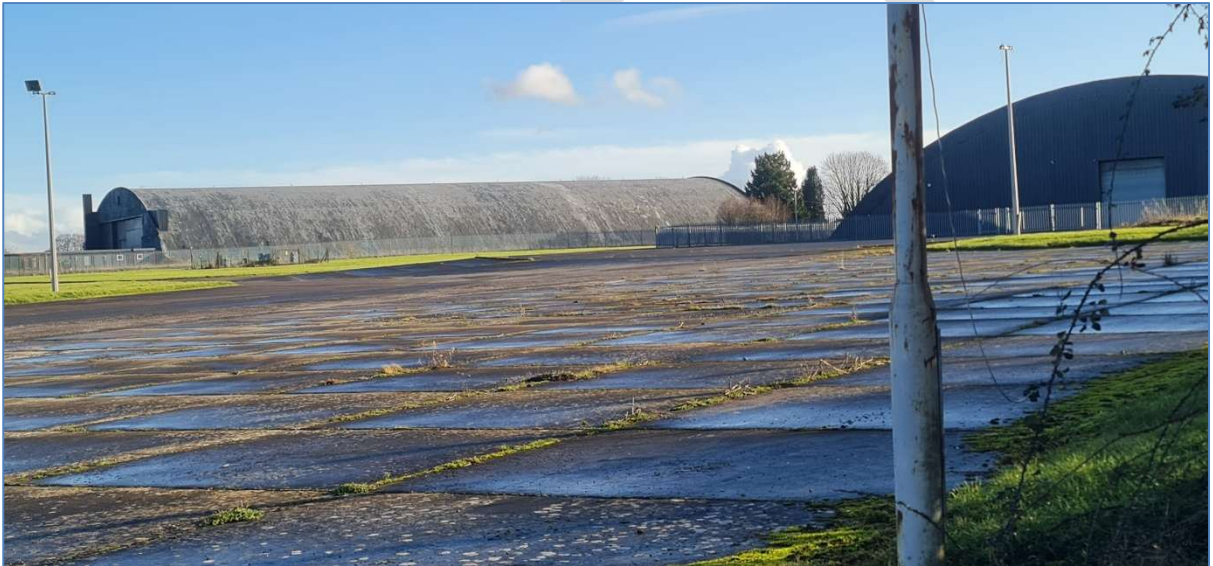
Plate 9 Hangar 19, left, in January 2026, with Hangar 20 to the right
