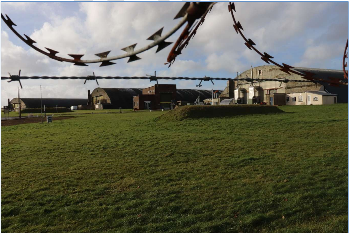
Plate 21 The three L Type hangars at Priddle's Site 4, in January 2026, seen from Doncombe Lane looking west, showing the retained boiler room and crew office annexes and smaller sliding doors.
