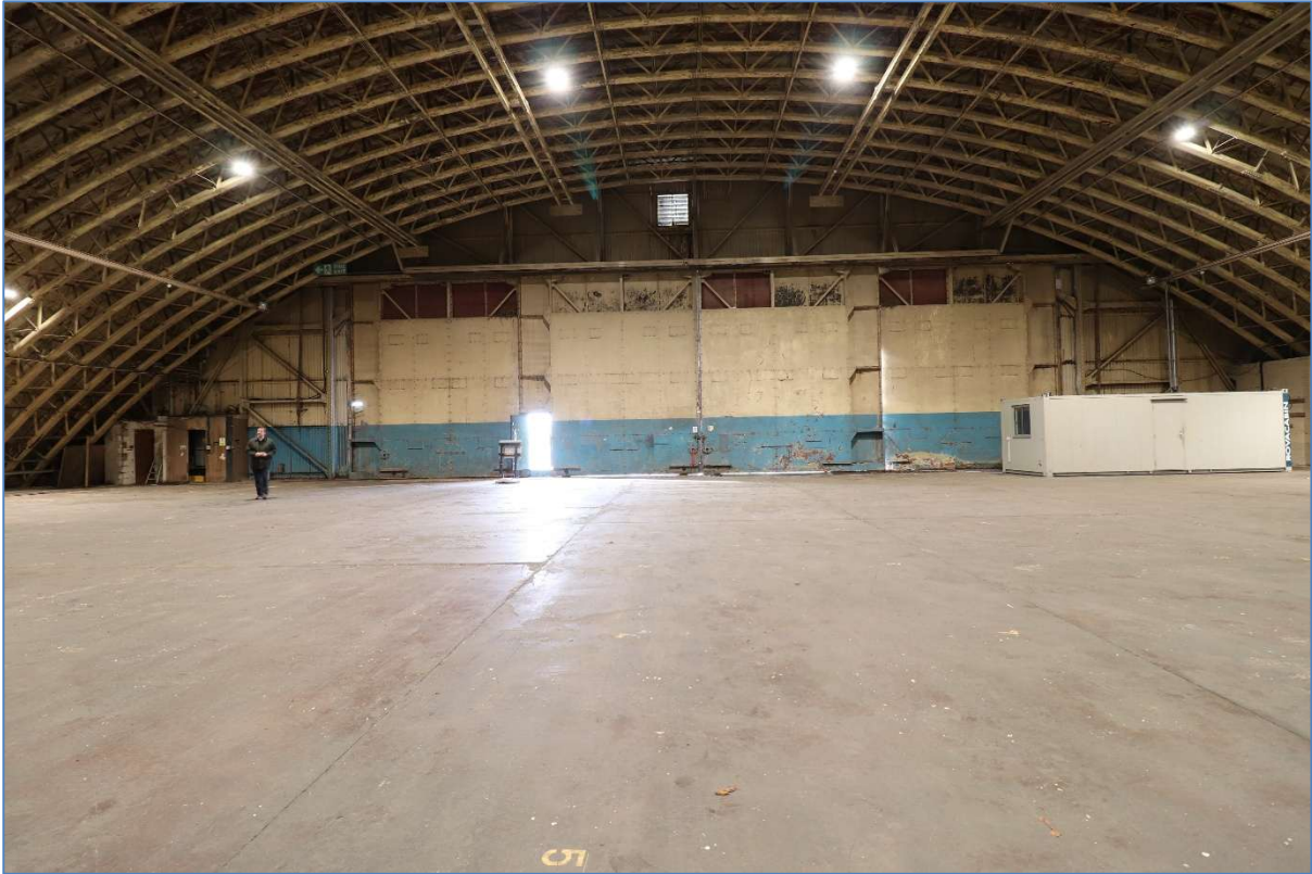
Plate 12 The interior of Hangar 18, in January 2026, showing the larger sliding doors at the western end.
