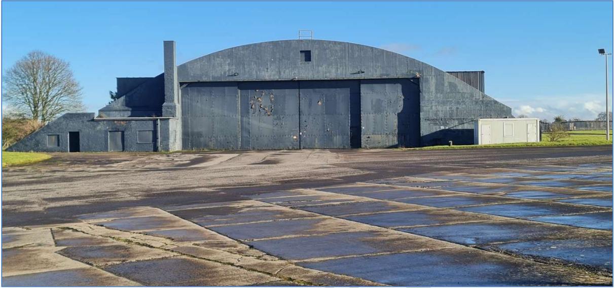
Plate 7 Hangar 18 in January 2026, showing the added 'ears' which allowed wider opening of the doors
