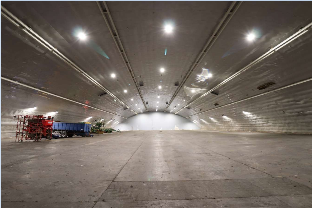
Plate 18 Hangar 20, in January 2026, looking south, showing the wall inserted in front of the retained southern sliding doors and the panels covering the roof struts.
