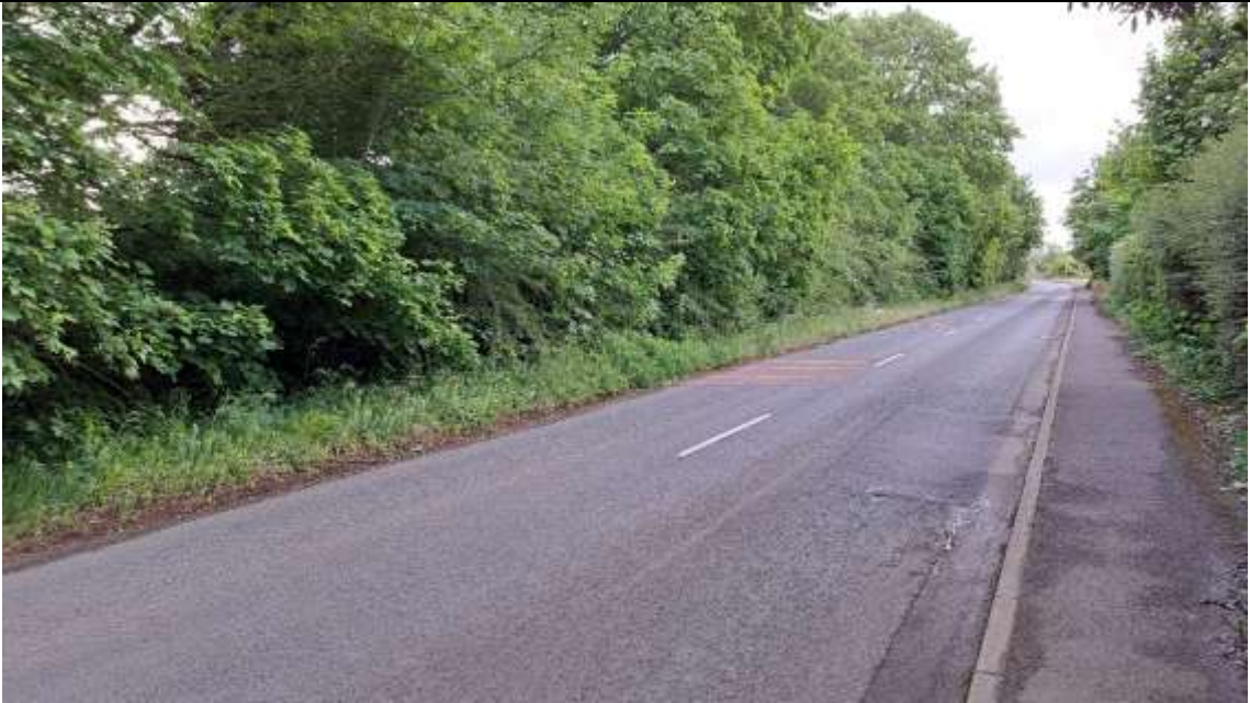
View along tree lined site frontage at highway at southern end of site. Photo taken from southern side of highway looking north-east. June 2026.
