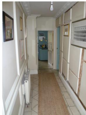
Entrance Hall looking north
