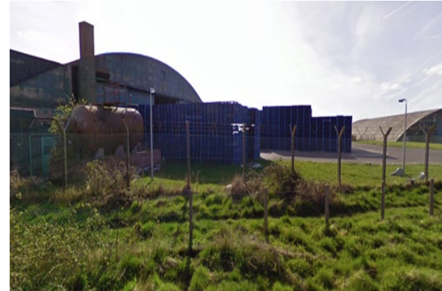
2 - High level floodlighting and column mounted lanterns within the existing Site
