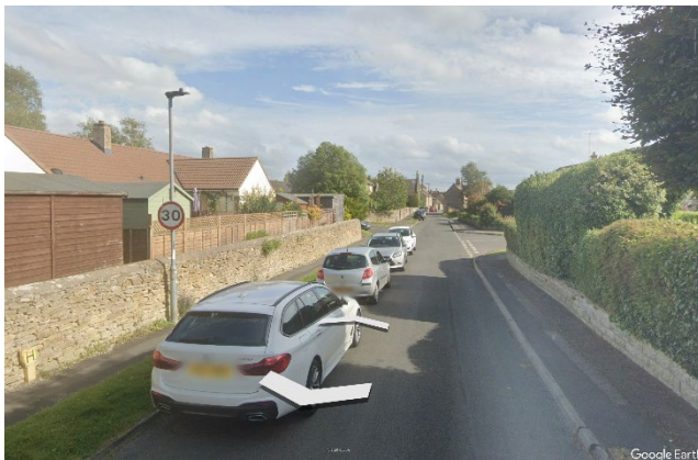
3 - Column mounted LED lanterns to roadways entering Colerne Village (Google Earth)
