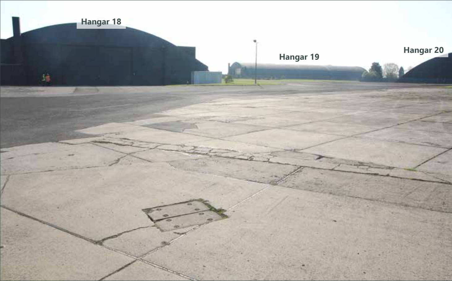
CV.I - View within site from north west corner
