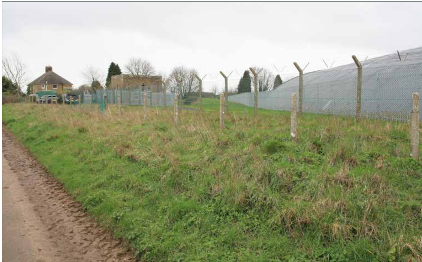
CV.G - Site eastern boundary, Hanger 19, sub station and residential properties
