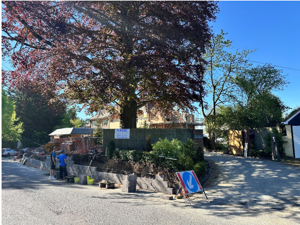
Figure 1: Inner blockwork being laid.
