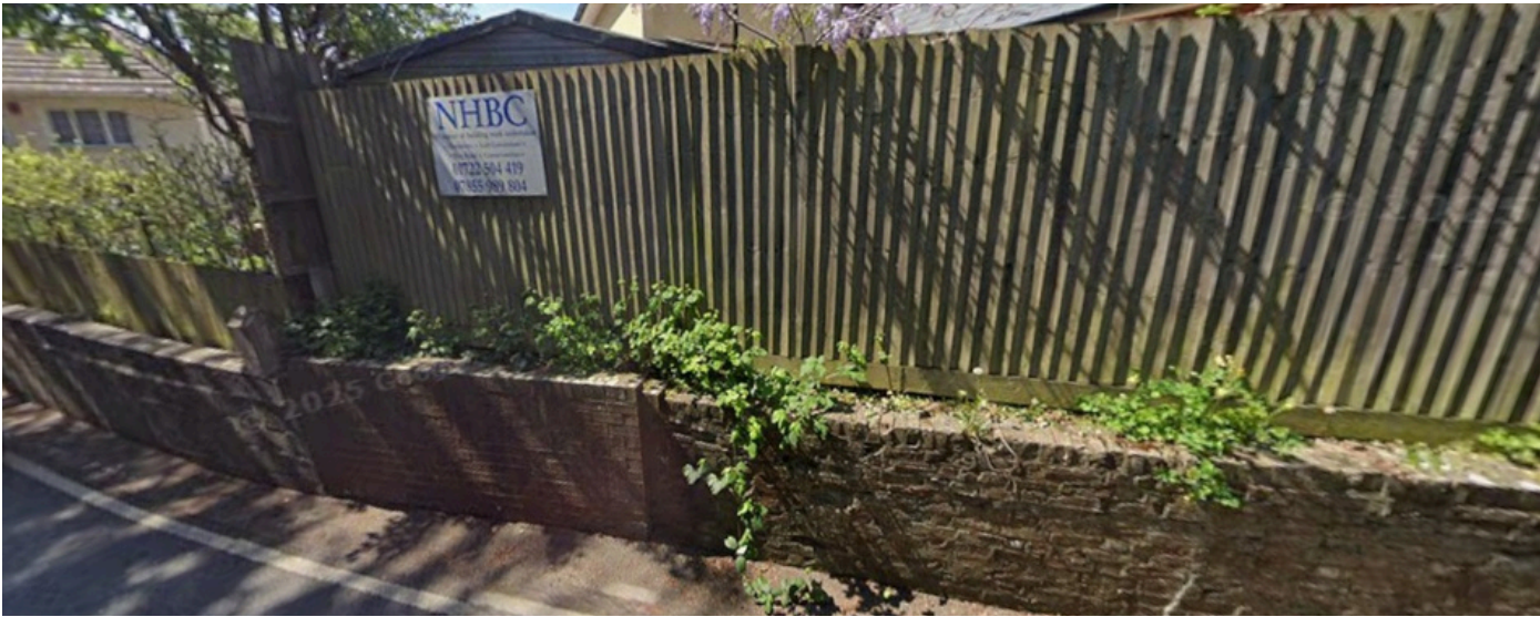
PREVIOUS EXISTING WALL AND FENCE VIEW D
