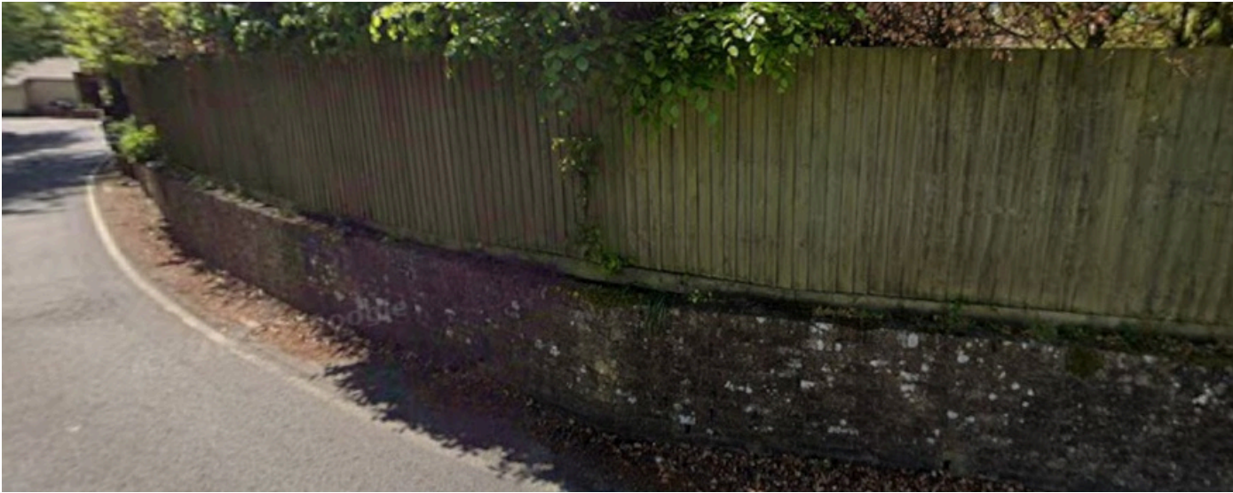
PREVIOUS EXISTING WALL AND FENCE VIEW C
