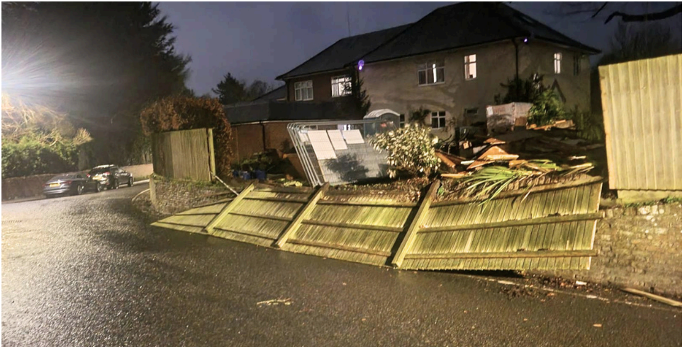
PREVIOUS EXISTING FENCE COLLAPSE AND ROAD CONTEXT
