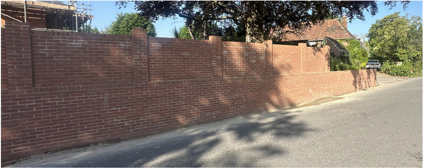
CURRENT EXISTING WALL VIEW B
