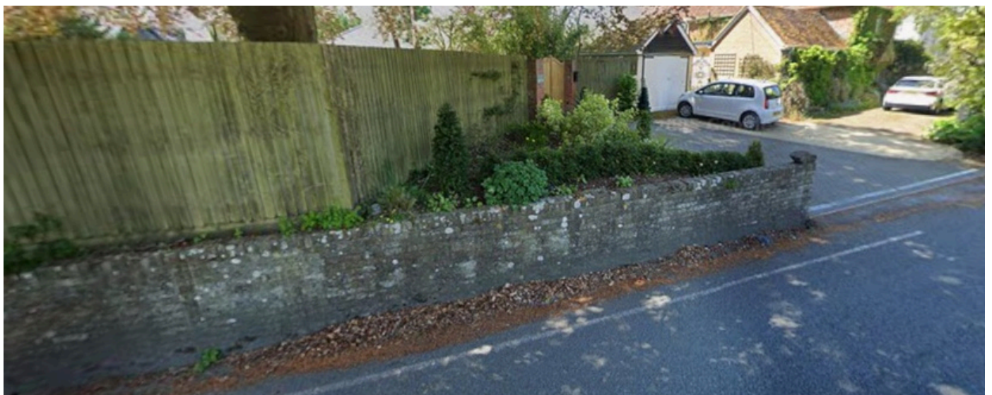
PREVIOUS EXISTING WALL AND FENCE VIEW A
