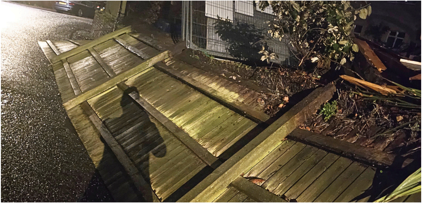
PREVIOUS EXISTING FENCE COLLAPSE
