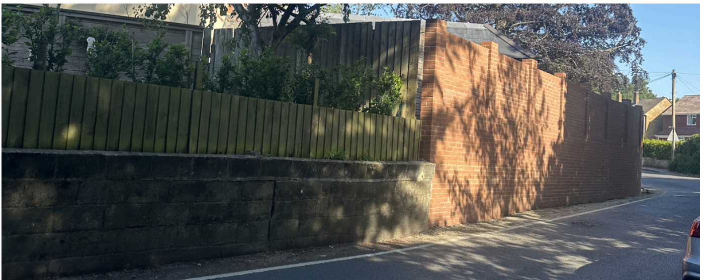
CURRENT EXISTING WALL VIEW D
