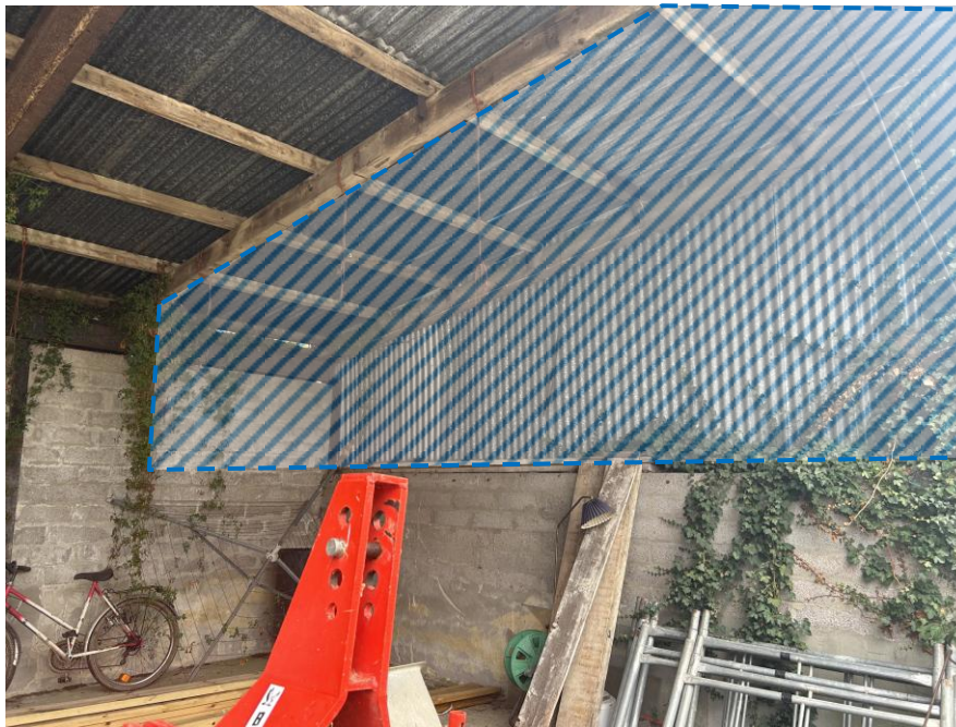
Fig 30: This area of the barn to the south of the new dwelling will be enclosed to provide a void space for brown long-eared bats.
