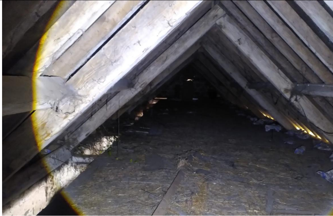
Fig 7. The interior of the barn had an empty roof void which was a single, continuous space. Photo taken 20 th April 2026.
