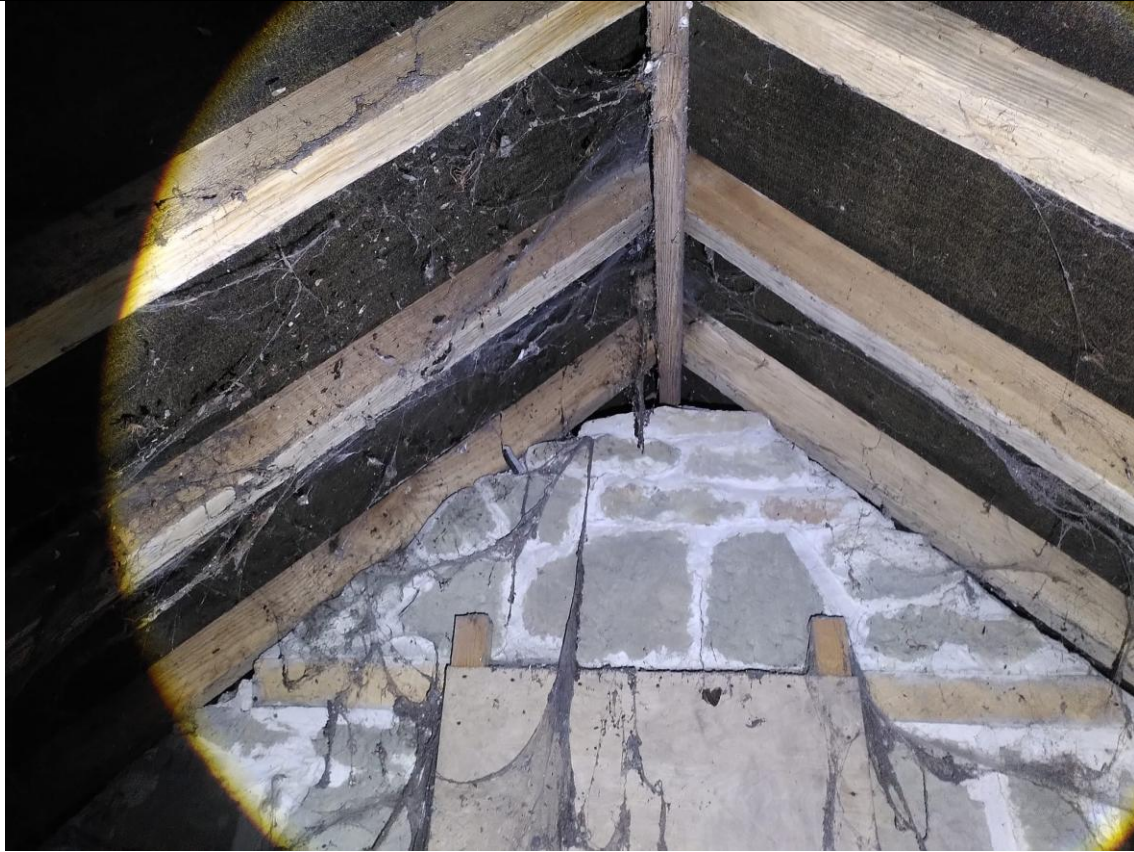
Fig 19. An internal wall at the southern end approximately 30 cm from the external wall. Photo taken 20 th April 2026.
