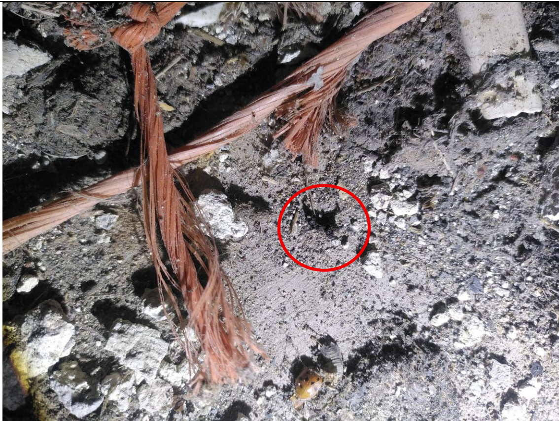
Fig 20. Example of bat dropping found on the floor of the barn roof void.
