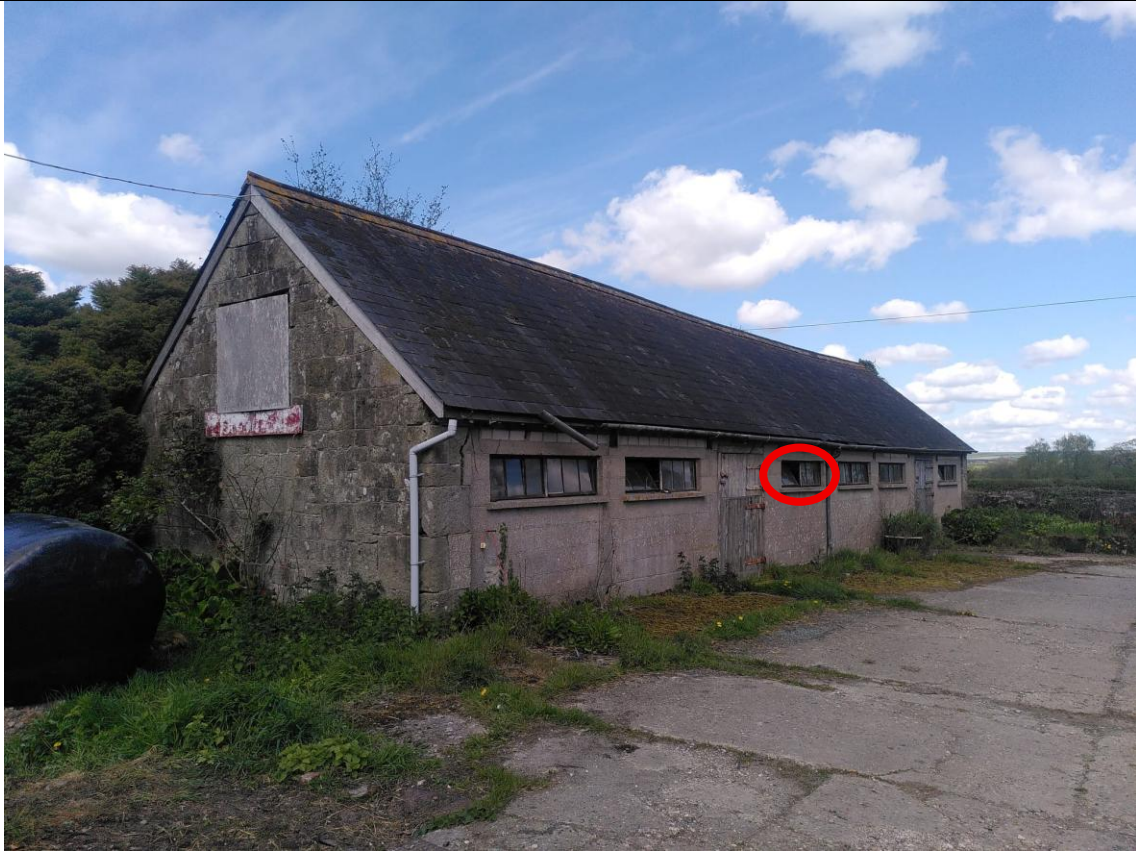
Fig 22. At 2217 surveyor two recorded one common pipistrelle emergence from the centre window of the eastern elevation.
