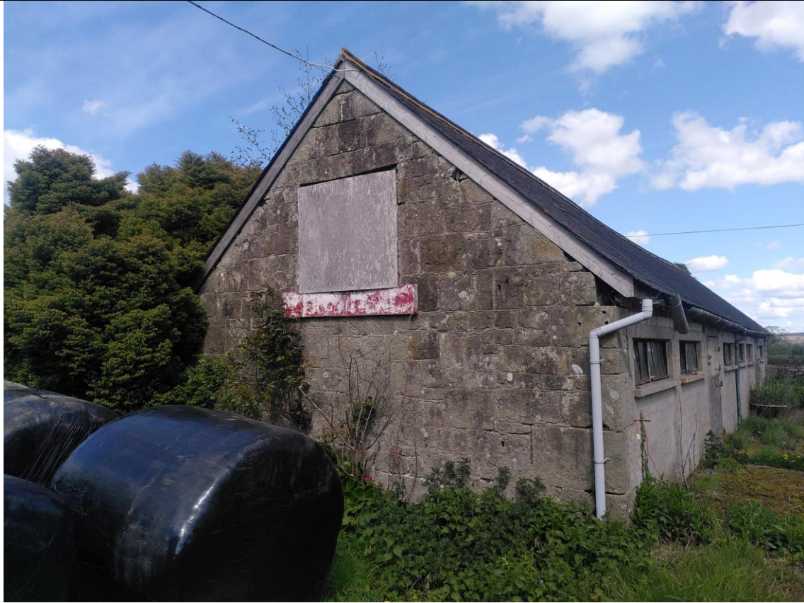
Fig 11. The southern elevation was a gable end and had a boarded window in the centre. Photo taken 20 th April 2026.
