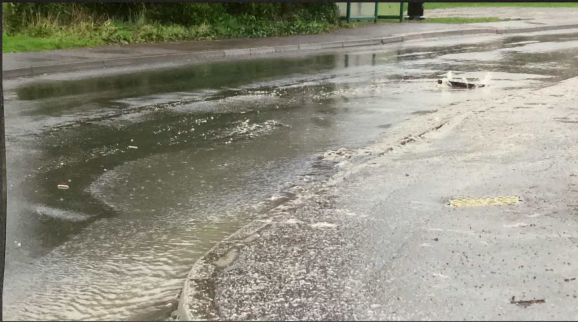
Sewage flowing down woodcock rd
