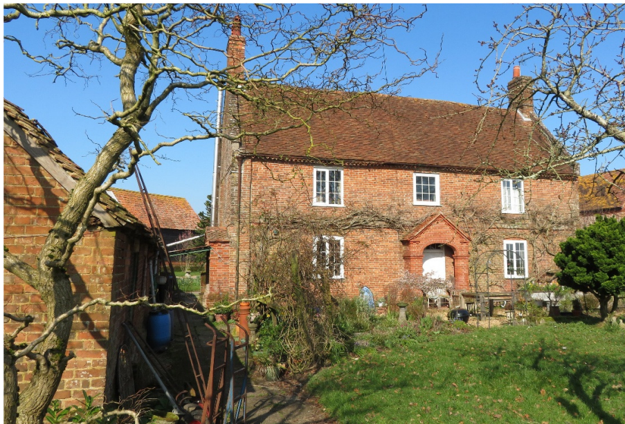
Photo viewing present Rear of Property from Back Garden (Camera Facing North)
