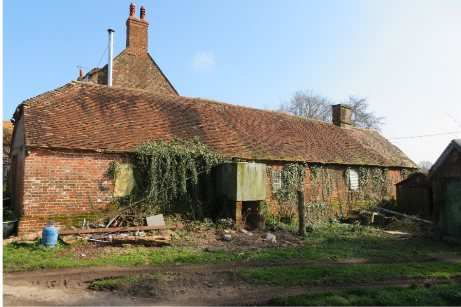
Photo viewing present Side of Outbuilding from Drive (Camera Facing East)
