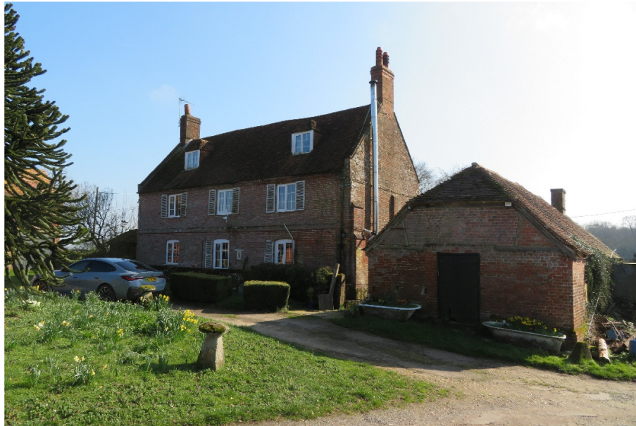
Photo viewing present Frontage / Side of Property & Outbuilding from Drive (Camera Facing South East)
