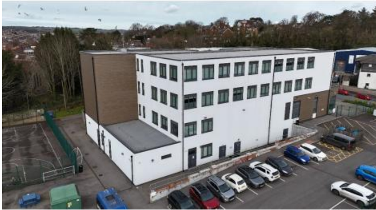
East and South elevations of the building showing rear service wing
