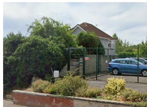
Tollgate Road gated footway
