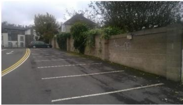
Plate 10: Car park and wall supporting vegetation (south-eastern boundary)
