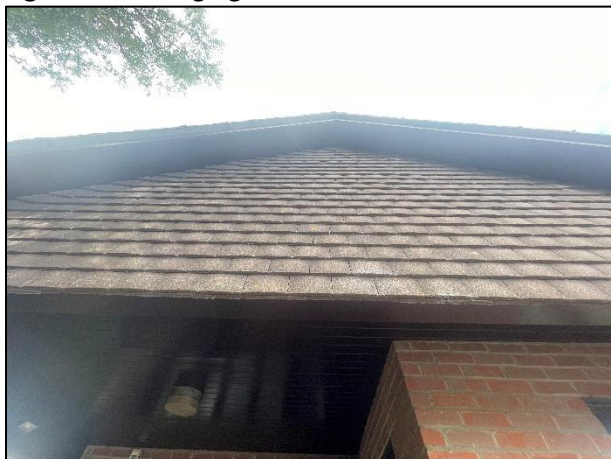
Figure 4.10 Hanging tiles on east elevation of Building B1
