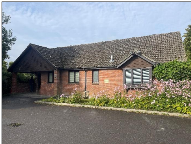
Figure 4.10 Hanging tiles on east elevation of Building B1
