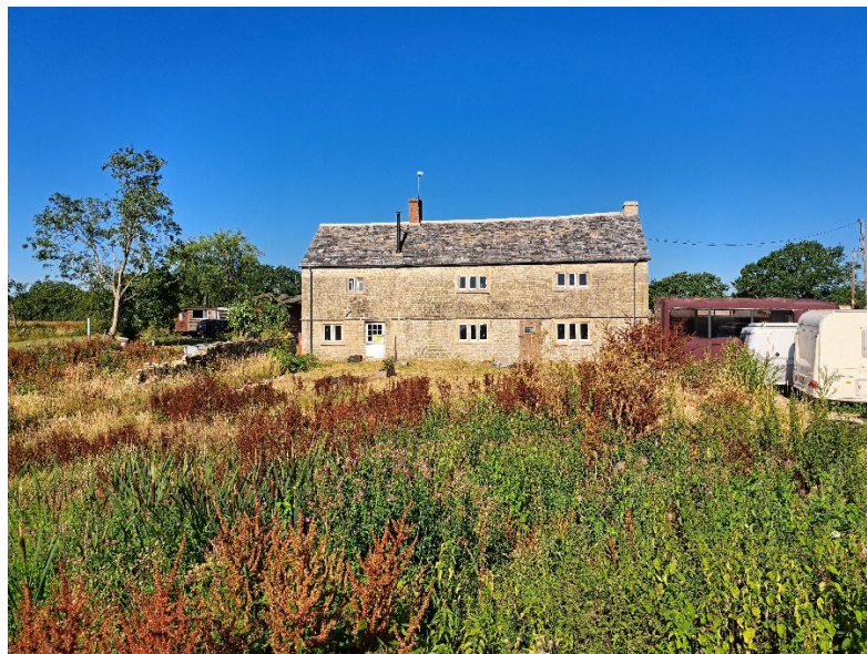
Main Farmhouse Renovation Upper Studley Farm, Swindon Road, Royal Wootton Bassett, SN4 8ET
