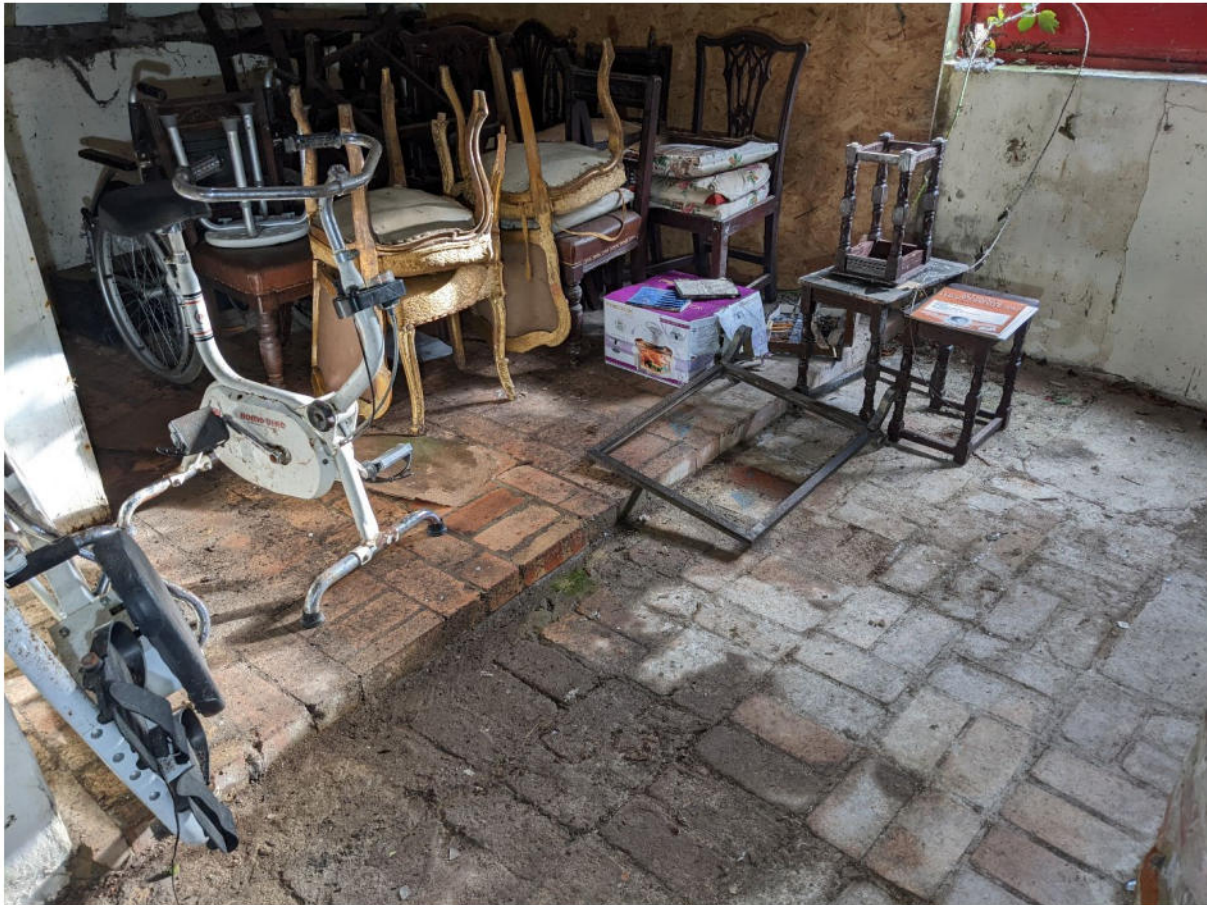
Image 2- 2022, Southeast end of Barn / Hall showing Fletton brick pavers.
