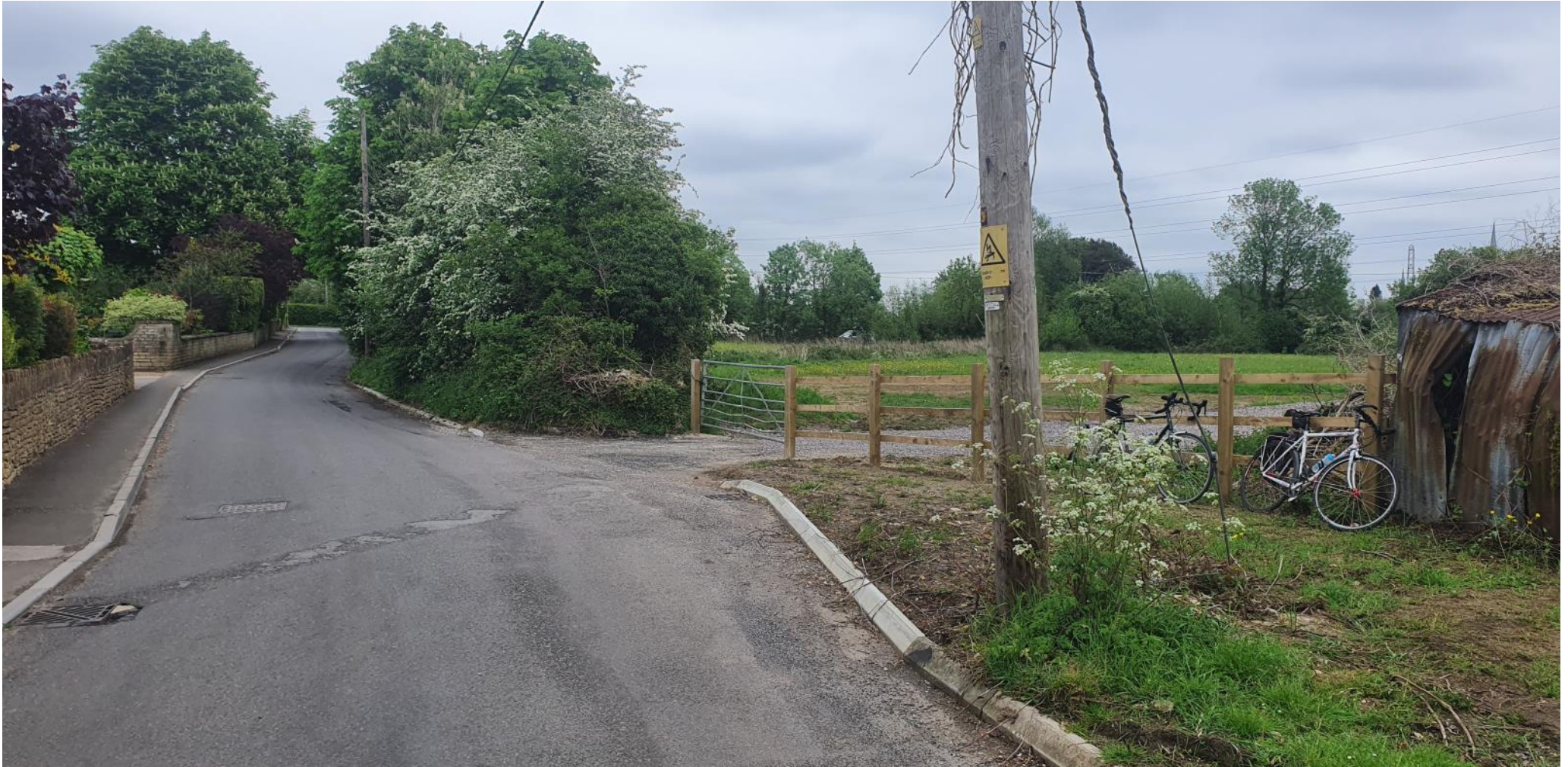
Photo 1: The existing field gate access to the application site from First Lane, Whitley. The Council recently completed works to a surface water culvert that crosses First Lane into a drainage ditch in the application site.
