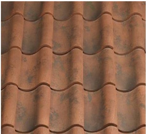
Fig 3: Clay Roof Tiles
