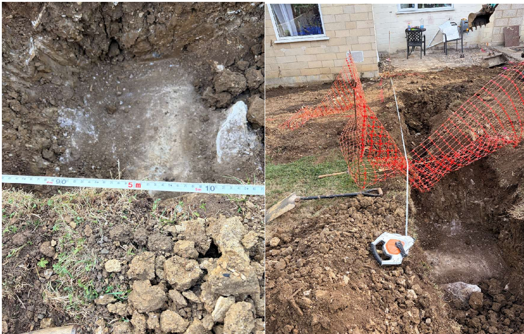
Culvert 5Mtrs from existing extension and 700mm below Ground level
