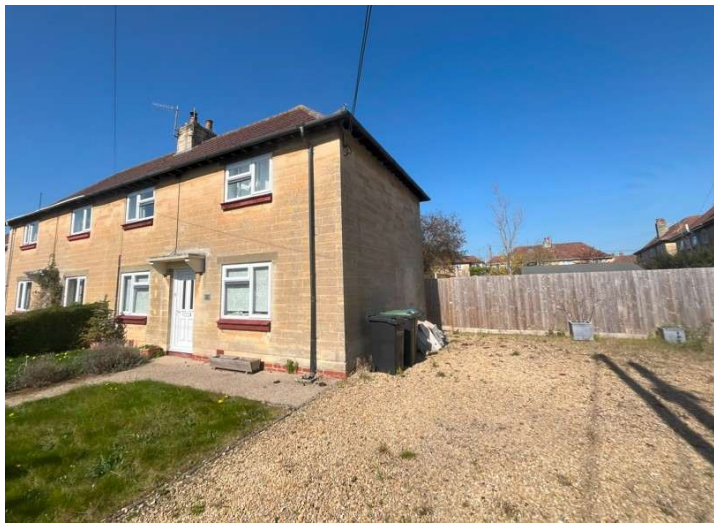
Photograph 2 - View of front garden of 2 North End and side gravel area.
