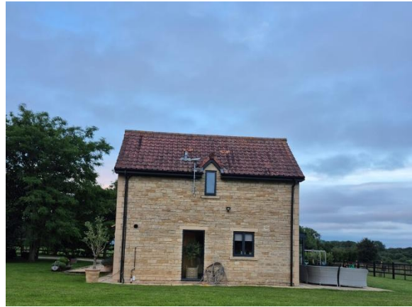
Photo 2 – View of building 1 from the position of surveyor 1.
