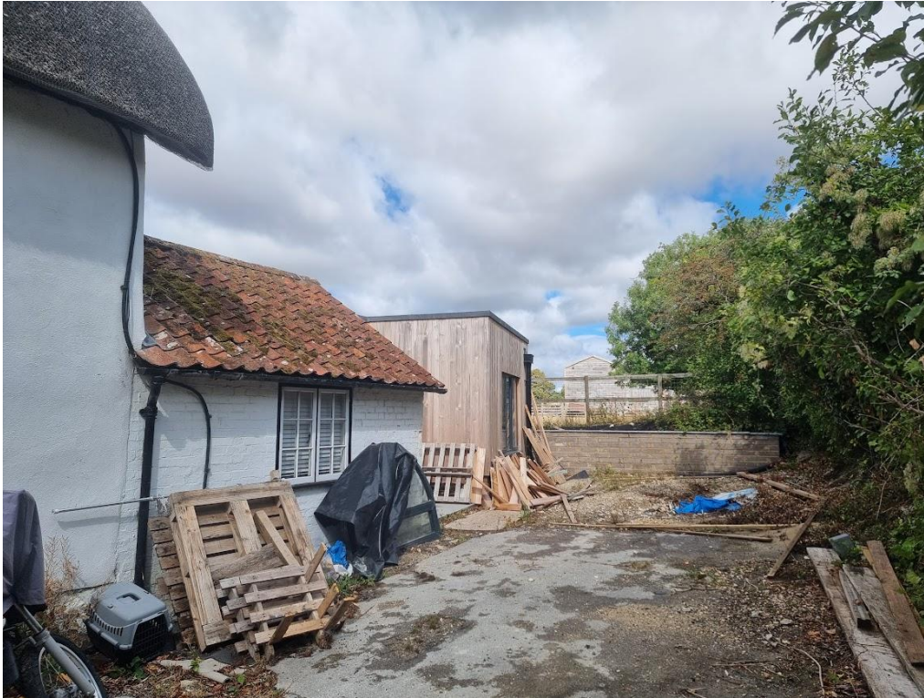
Figure 3: The small single-storey gabled addition at the northern end of the cottage, retaining its clay pantile roof. Beyond is the recently constructed annexe, of brick plinth, timber cladding and flat roof.
