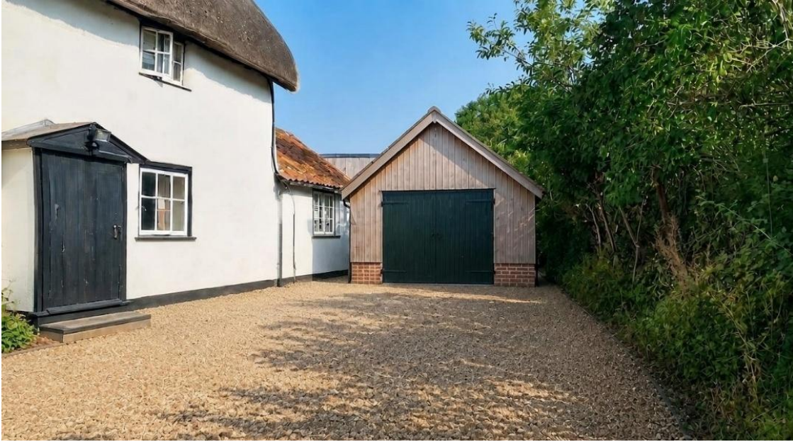
Figure 9: Three-dimensional visualisation of the proposed single-bay garage, showing the pitched gabled roof, vertical timber weatherboarding, brick plinth and boarded doors.
