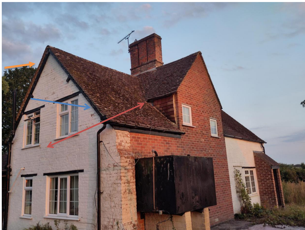
Figure 3: showing bat egress/ingress locations on the building (main dwelling)
