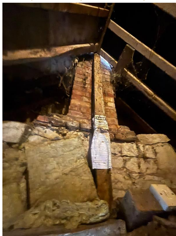
Photograph 4: showing a view of the chimney stack internally
