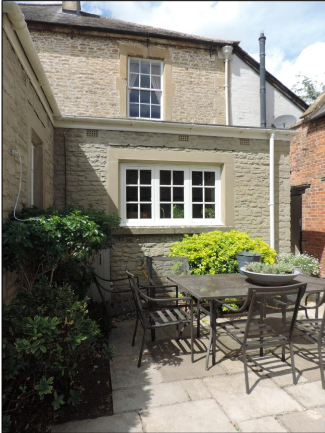
Photo 6 West facing view of window to be enlarged within 1980s Kitchen extension.
