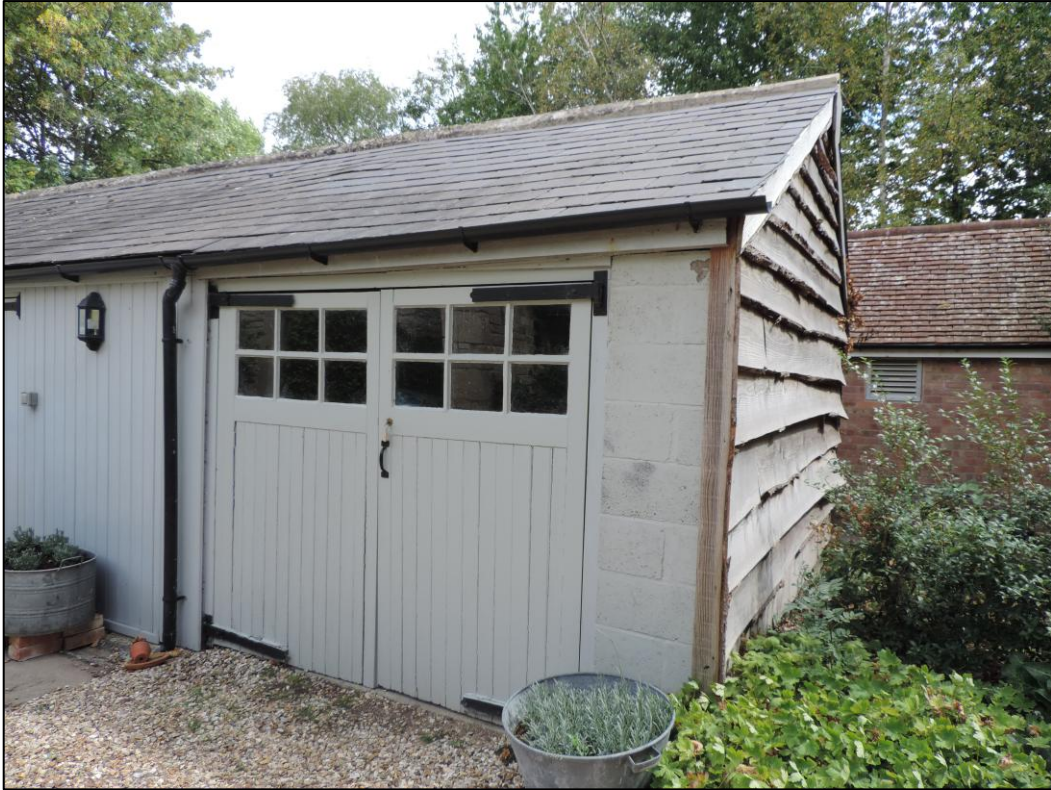
Photo 8 Northeast facing view of west elevation of modern concrete-block bay at the southern end of the Guest Annex / Studio.
