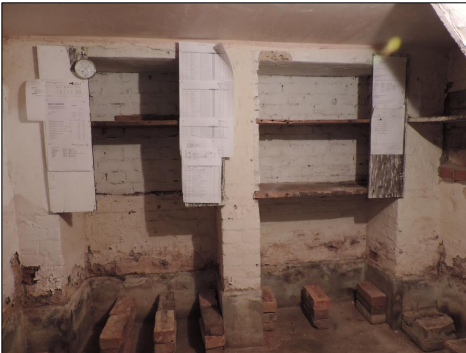
Photo 5 brick recesses against south wall of cellar. The height of these recesses corresponds to the raised ceiling height of the cellar noted to have occurred between 1949 and 1979.
