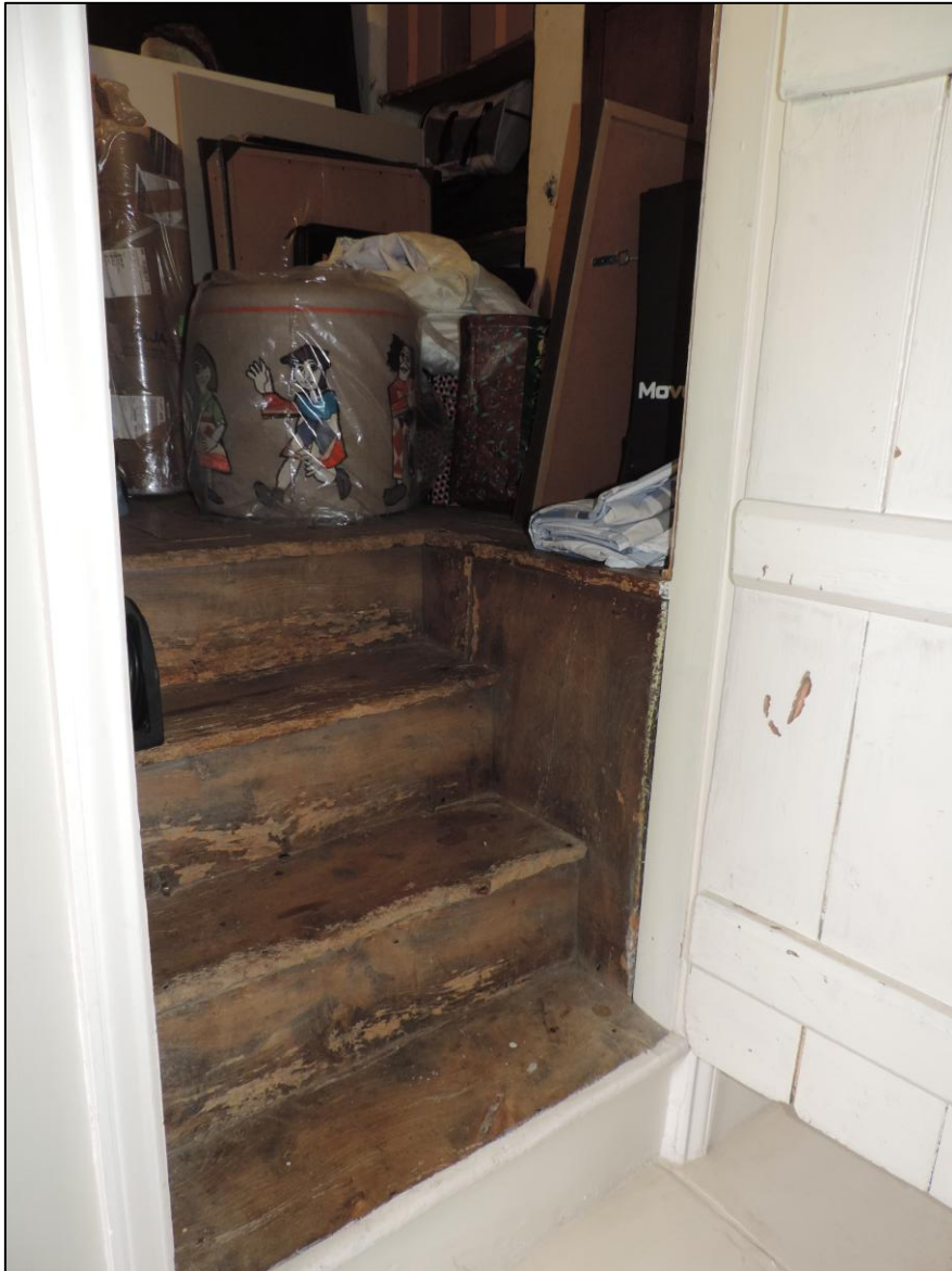
Photo 1 Restricted view of access from the north Reception Hall to mid 20 th century mezzanine above cellar.
