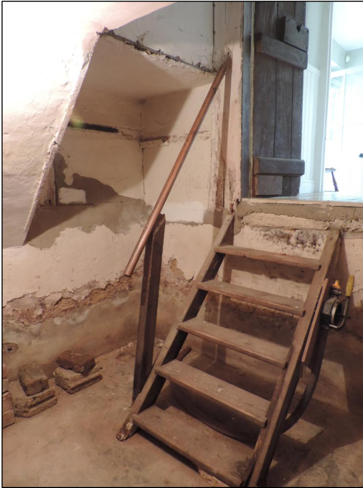
Photo 4 Steps leading down to cellar from north passageway.
