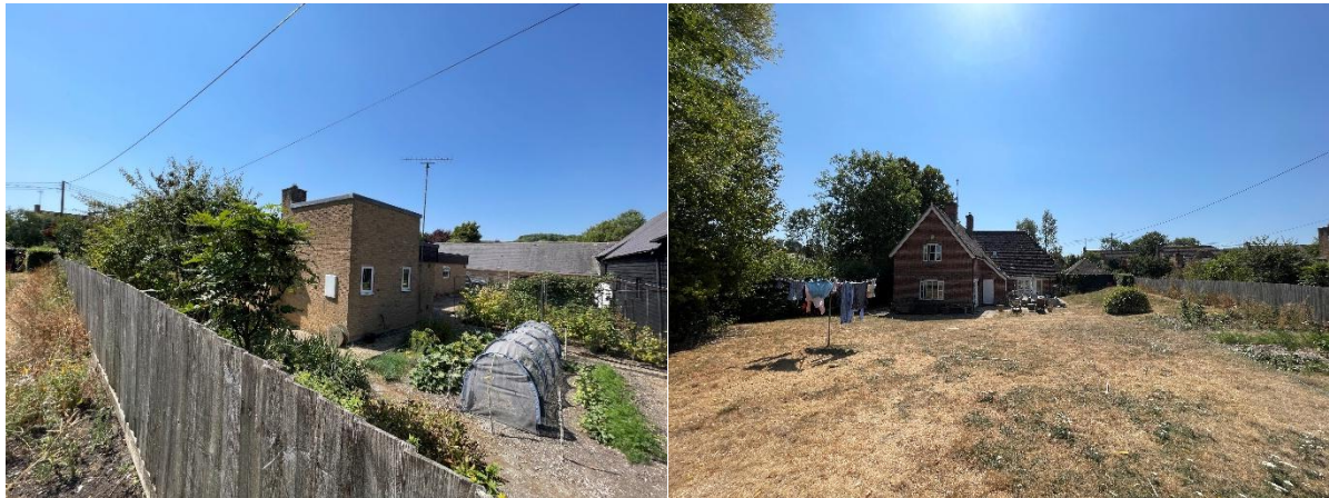
View of Sylvanus from Barn Lodge and north elevation of Barn Lodge, looking south
