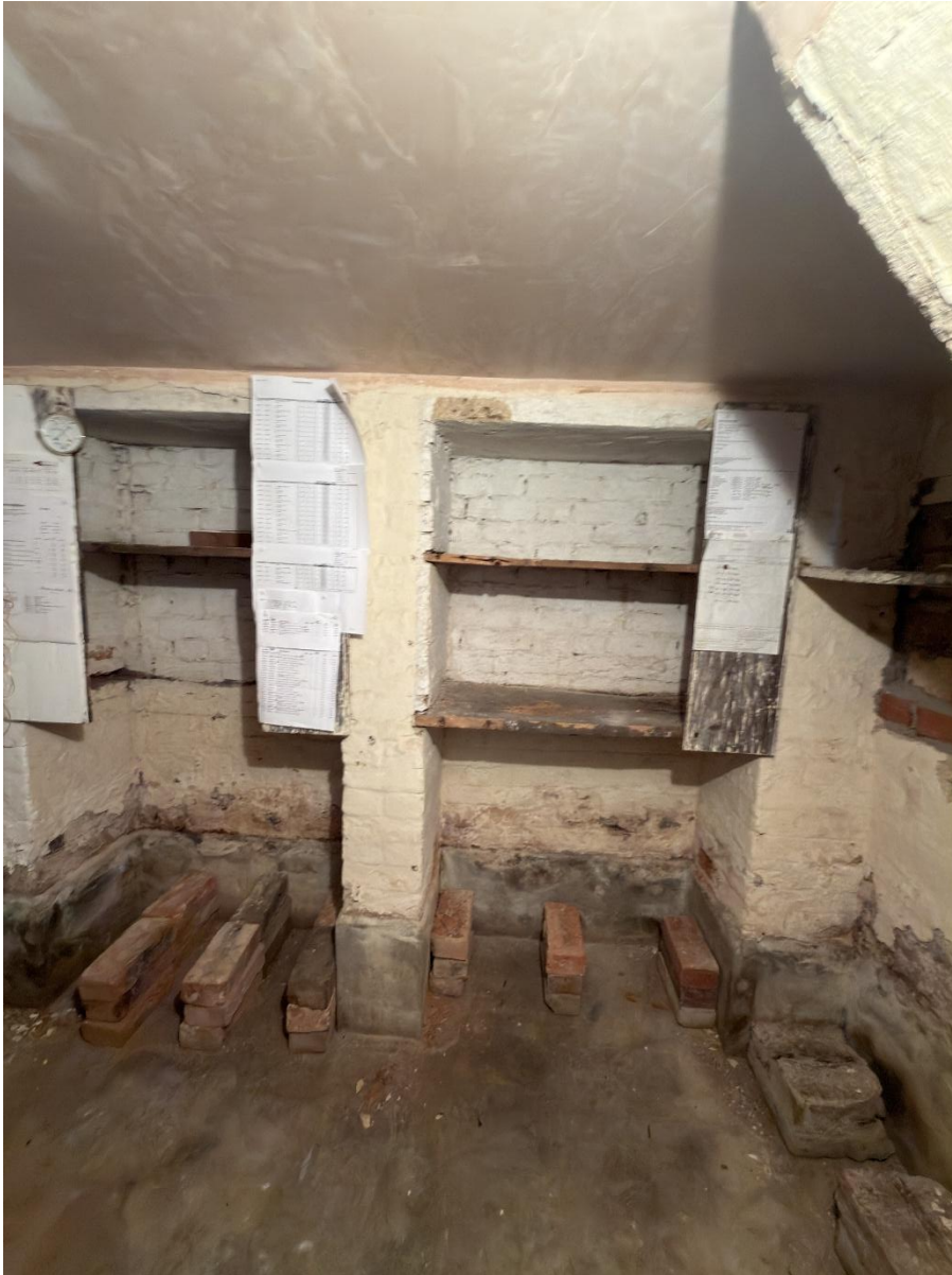
Figure 3. Existing kitchen cellar to be waterproofed and covered at kitchen floor level
