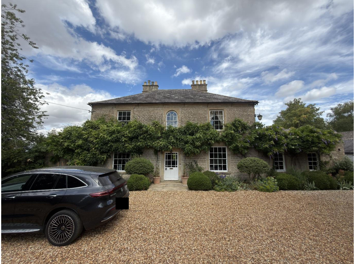
Figure 1. Front South facing elevation of Northfield House
