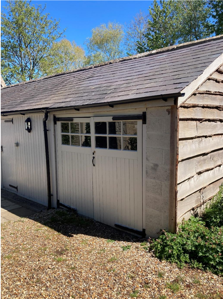
Figure 5. Blockwork garage extension (area C).
