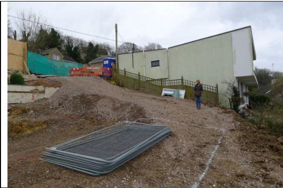
Plate 1 – Ramp down to site.
