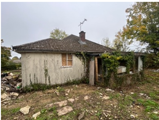
Photo 5: Western extent of bungalow within flat roofed boot room.
