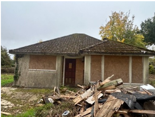
Photo 3: Front north-facing elevation of bungalow and rubble pile.
