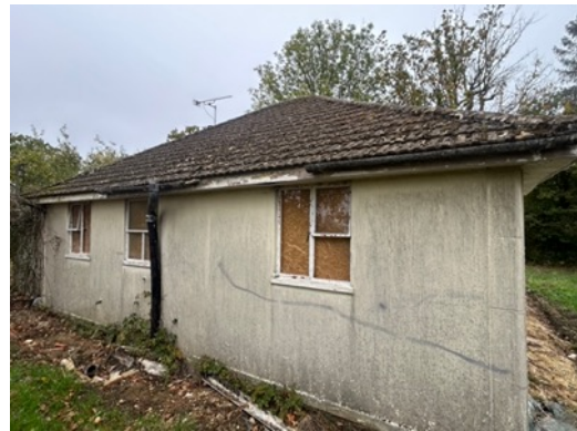
Photo 4: South-facing elevation and timber boarded windows.
