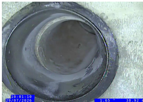
14, 00:08:49, 38.94 m Junction at 2 o'clock, 150mm dia
