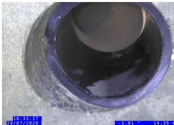
2, 00:02:43, 14.33 m Junction at 10 o'clock, 150mm dia
