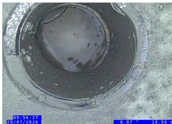
8, 00:04:09, 19.56 m Junction at 11 o'clock, 150mm dia
