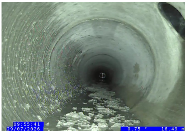
5, 00:03:23, 16.49 m Junction at 2 o'clock, 150mm dia
