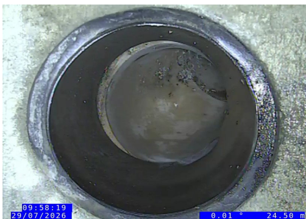
11, 00:06:01, 24.50 m Junction at 2 o'clock, 150mm dia
