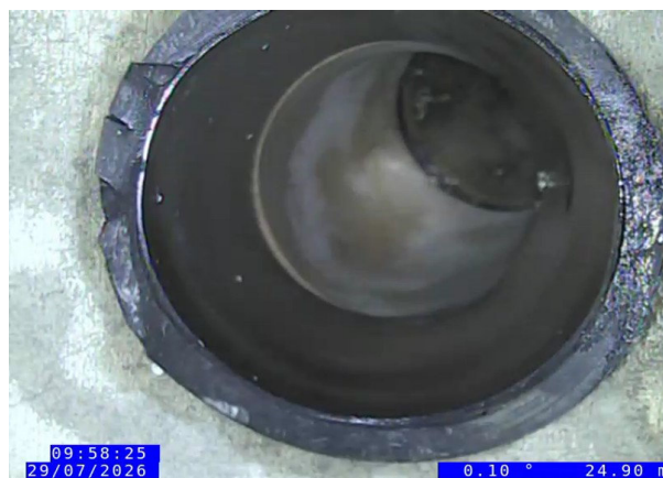
12, 00:06:05, 24.94 m Junction at 2 o'clock, 150mm dia
