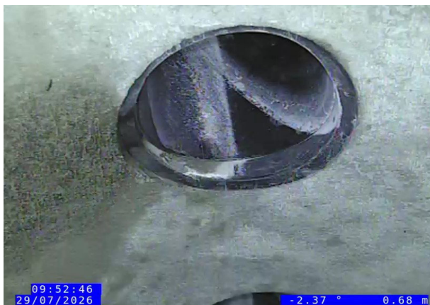
1, 00:00:32, 0.64 m Junction at 11 o'clock, 150mm dia
