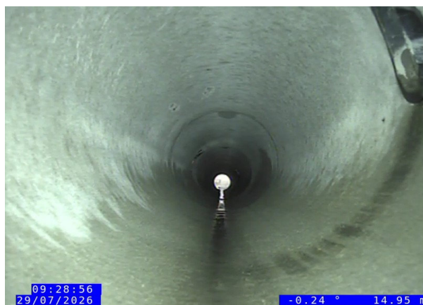
4, 00:03:36, 15.00 m Junction at 2 o'clock, 150mm dia
