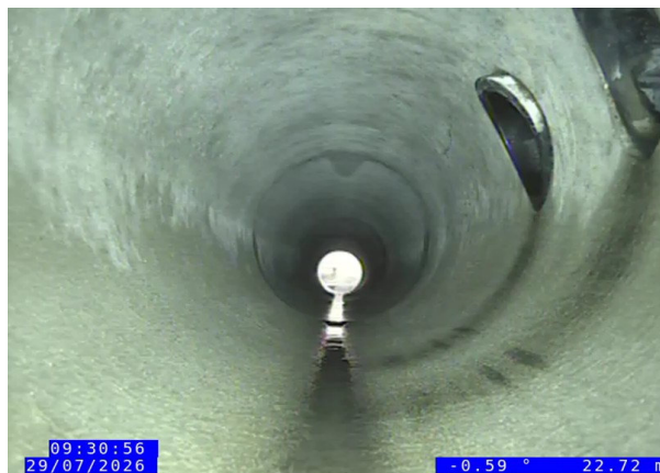
6, 00:05:36, 22.76 m Junction at 2 o'clock, 150mm dia
