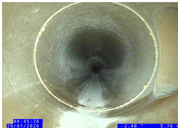
2, 00:02:00, 5.78 m Junction at 3 o'clock, 150mm dia
