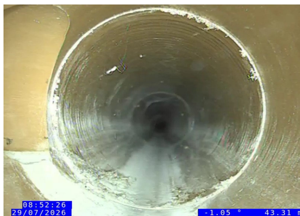
4, 00:08:57, 43.38 m Junction at 9 o'clock, 150mm dia
