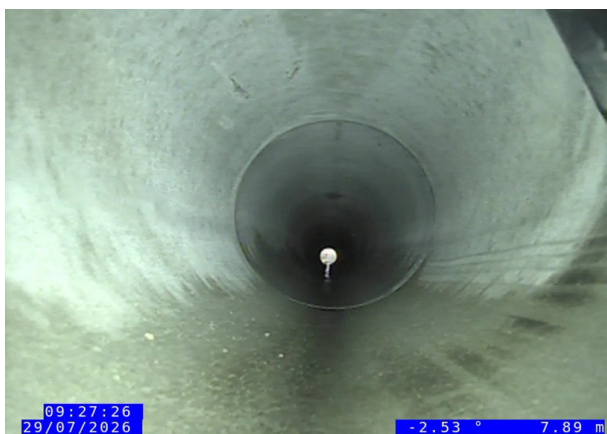
3, 00:02:06, 7.98 m Junction at 2 o'clock, 150mm dia
