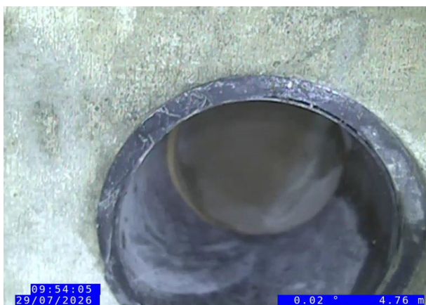
3, 00:01:47, 4.73 m Junction at 2 o'clock, 150mm dia
