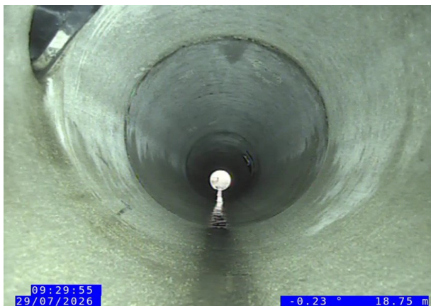
5, 00:04:35, 18.80 m Junction at 10 o'clock, 150mm dia
