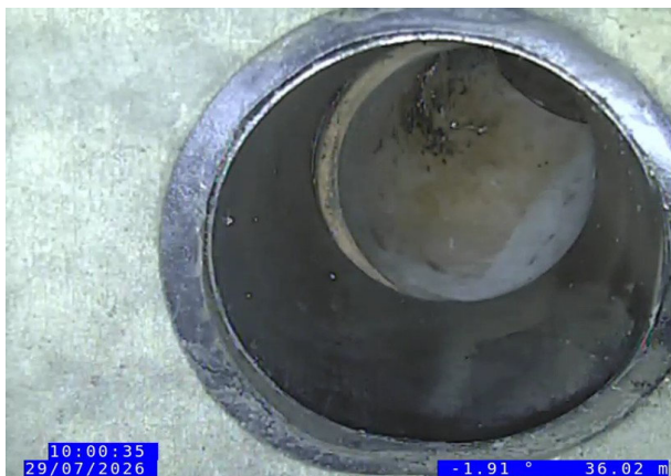
13, 00:08:14, 36.02 m Junction at 2 o'clock, 150mm dia
