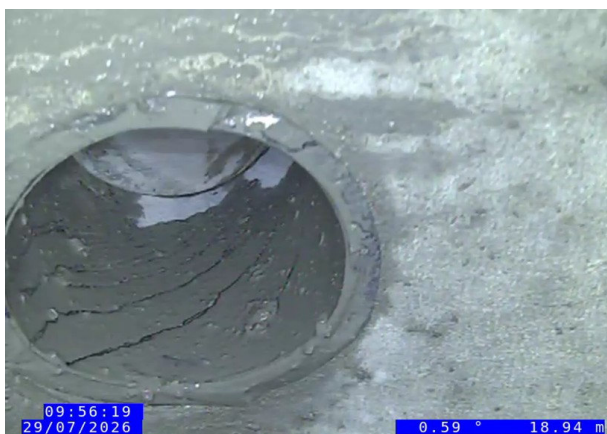
7, 00:04:01, 18.94 m Junction at 11 o'clock, 150mm dia
