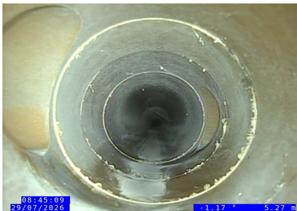
1, 00:01:43, 5.27 m Junction at 9 o'clock, 150mm dia
