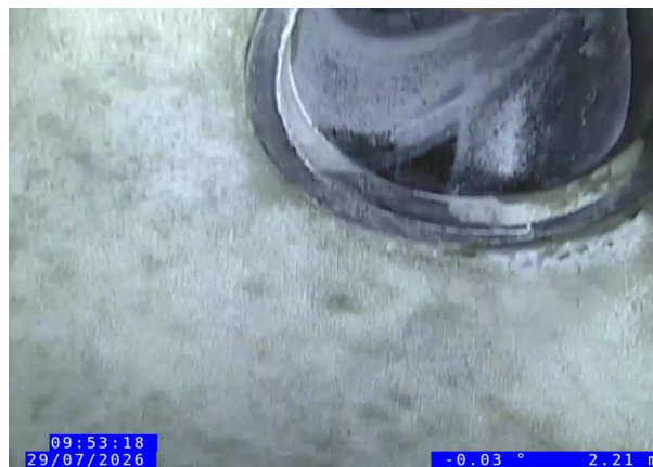
2, 00:01:00, 2.21 m Junction at 2 o'clock, 150mm dia
