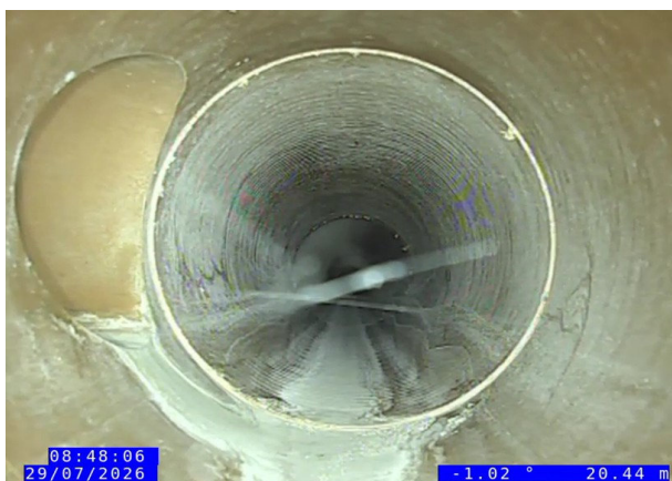
3, 00:04:40, 20.44 m Junction at 9 o'clock, 150mm dia
