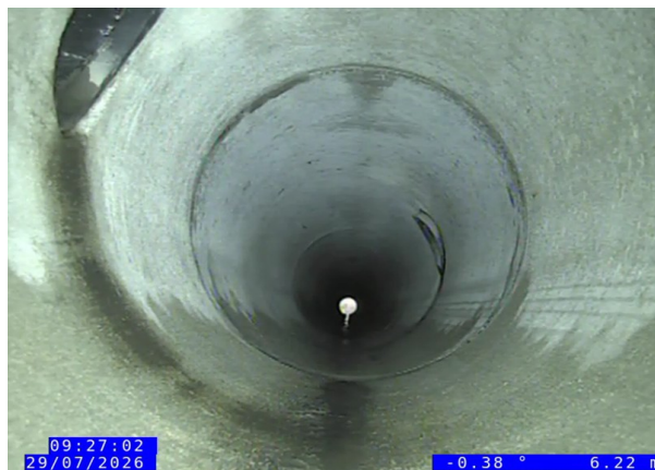
2, 00:01:42, 6.22 m Junction at 11 o'clock, 150mm dia
