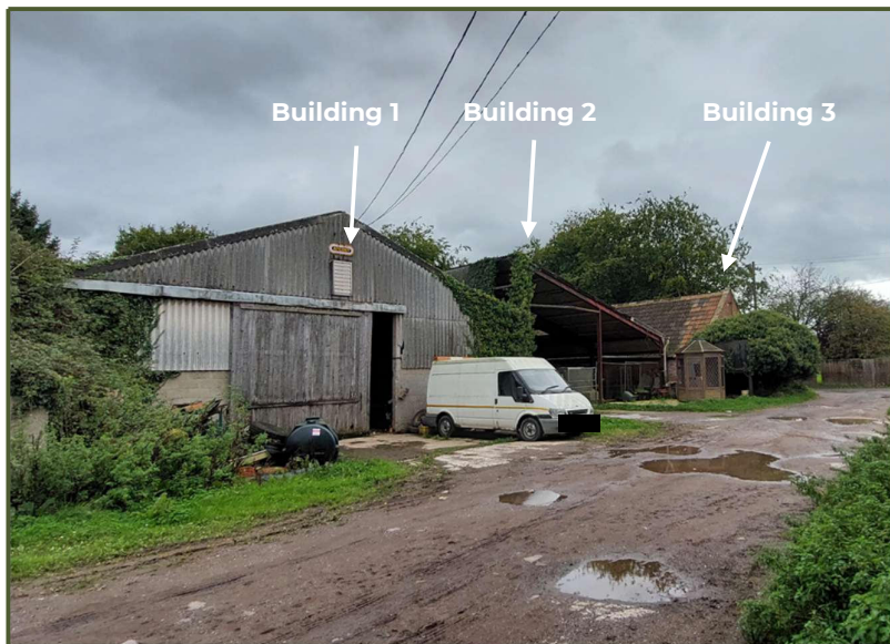
Fig 5 – Range of mid-20 th century farm buildings (buildings 1 & 2)
