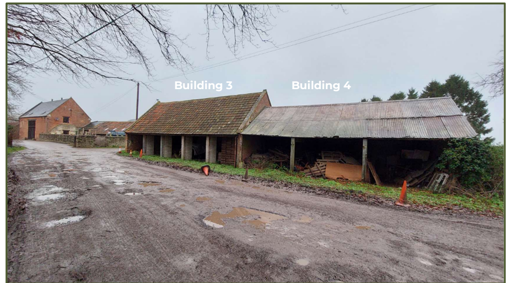
Fig 6 – Traditional building (building 3). The informal building 4 will be demolished
