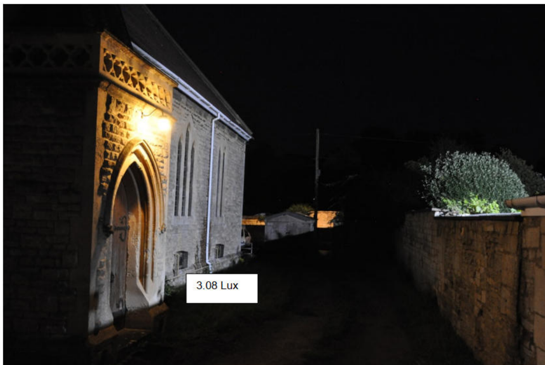
Plate 14 light spill on the south west side not used by bats
