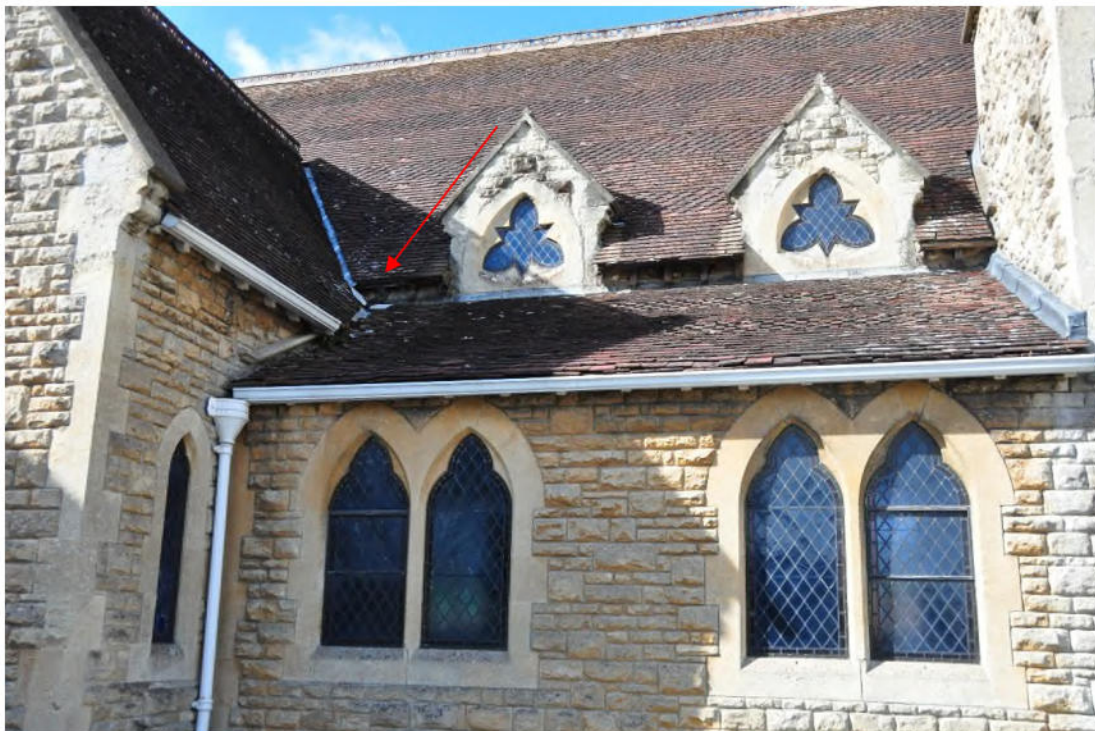
Plate 24 roof area to be re-roofed, long eared roost entrance in corner
