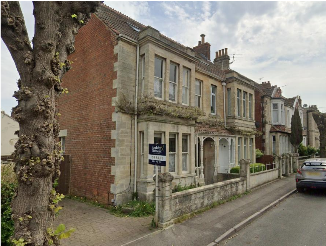
An example of a semi detached house in Trowbridge which demonstrates Stone front façade and brick to the rear/ sides. Note also the bay window design and integrated porch
