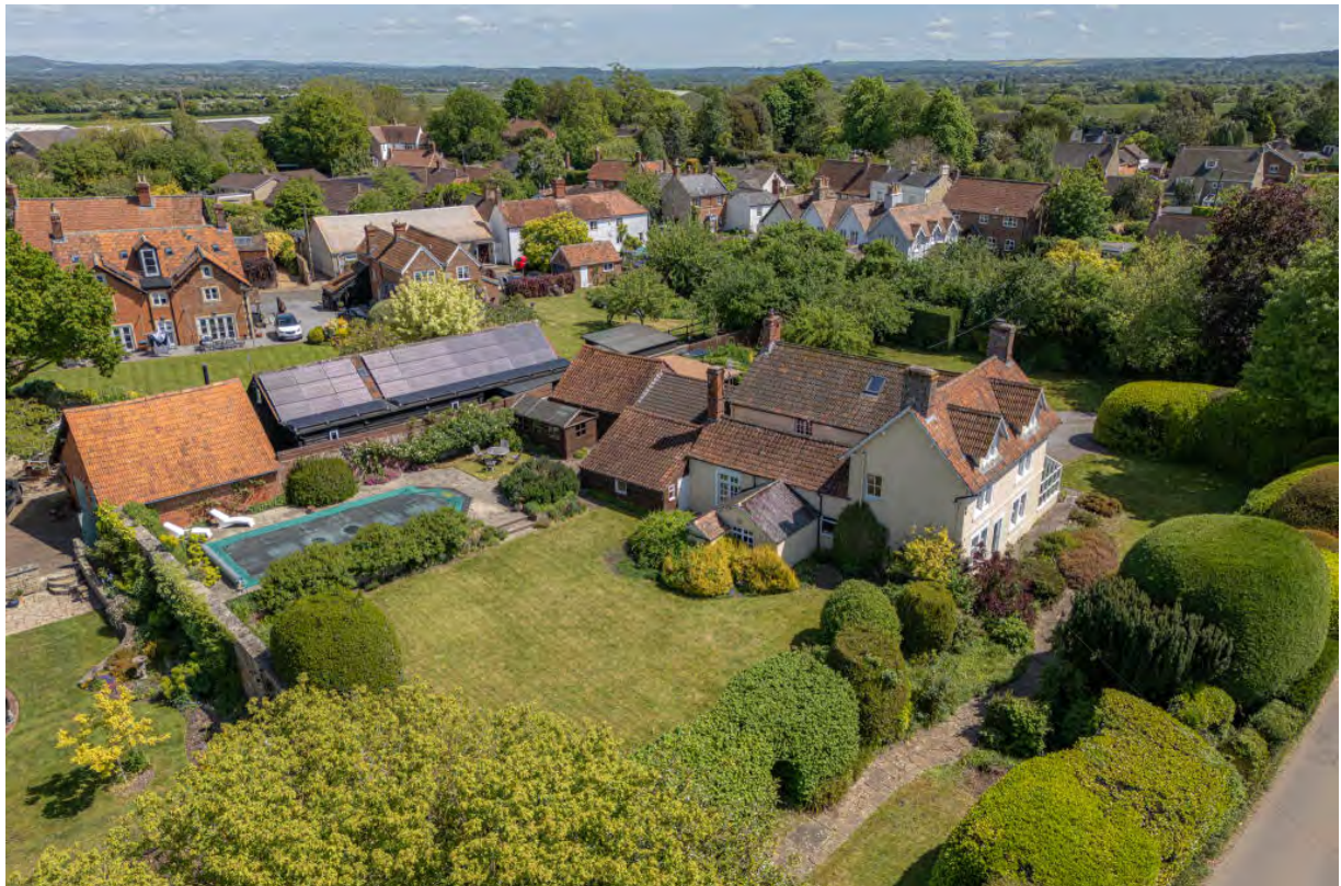
No 9 High Street and Solar Panels at Moorfield Lodge
