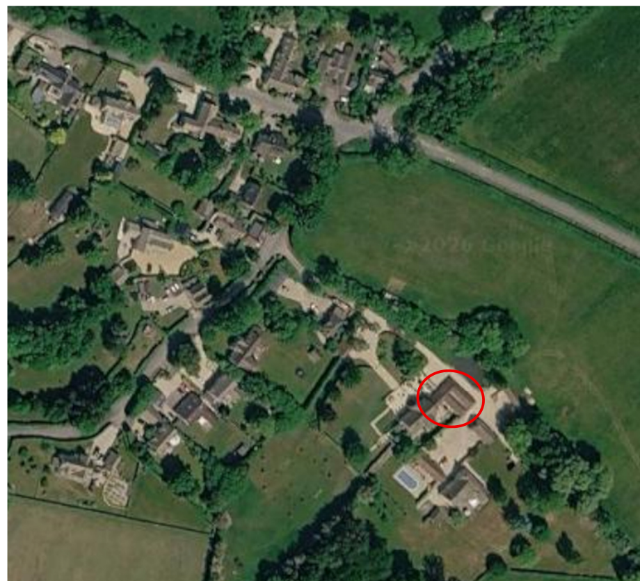
Figure 1. Aerial View of The Great Barn
