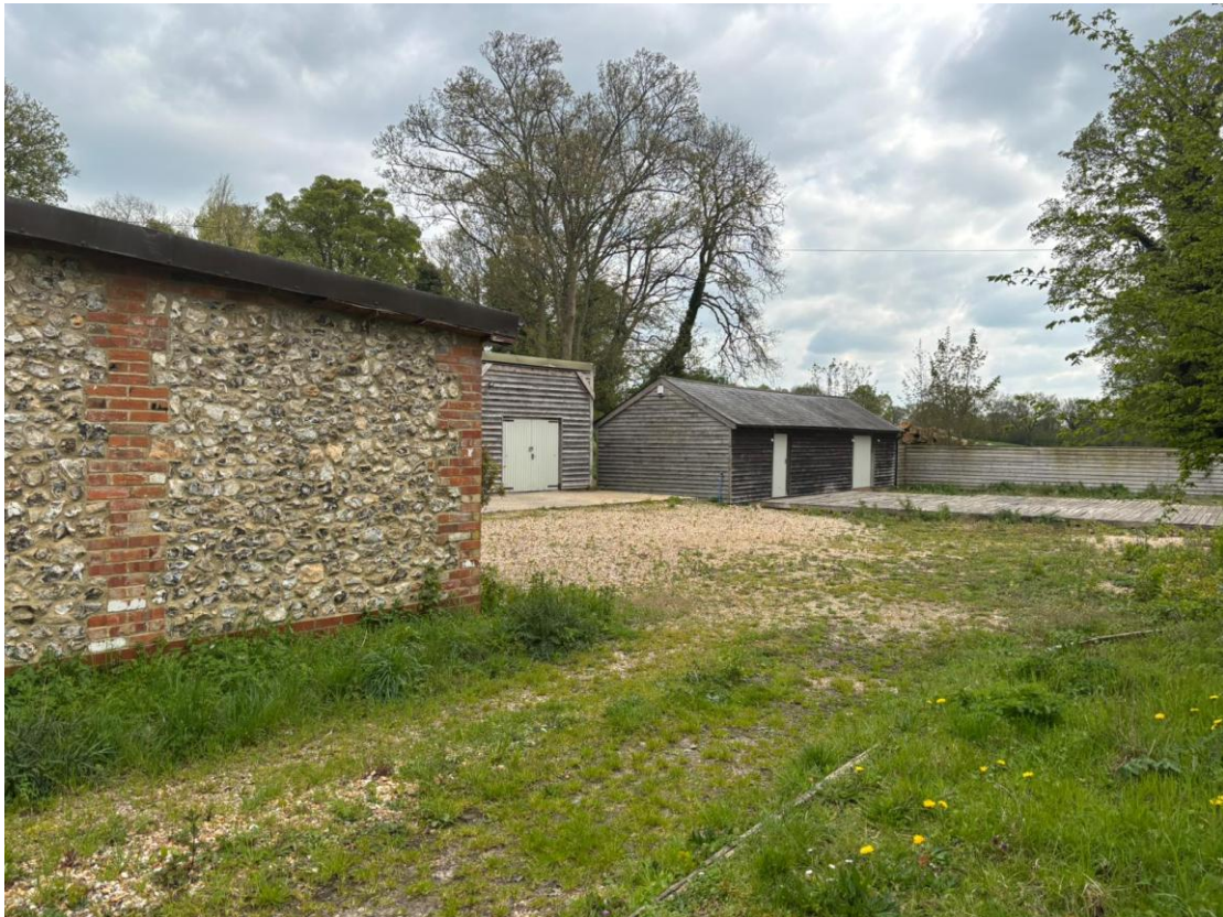
Figure 3 - Existing group of buildings and gravelled yard
