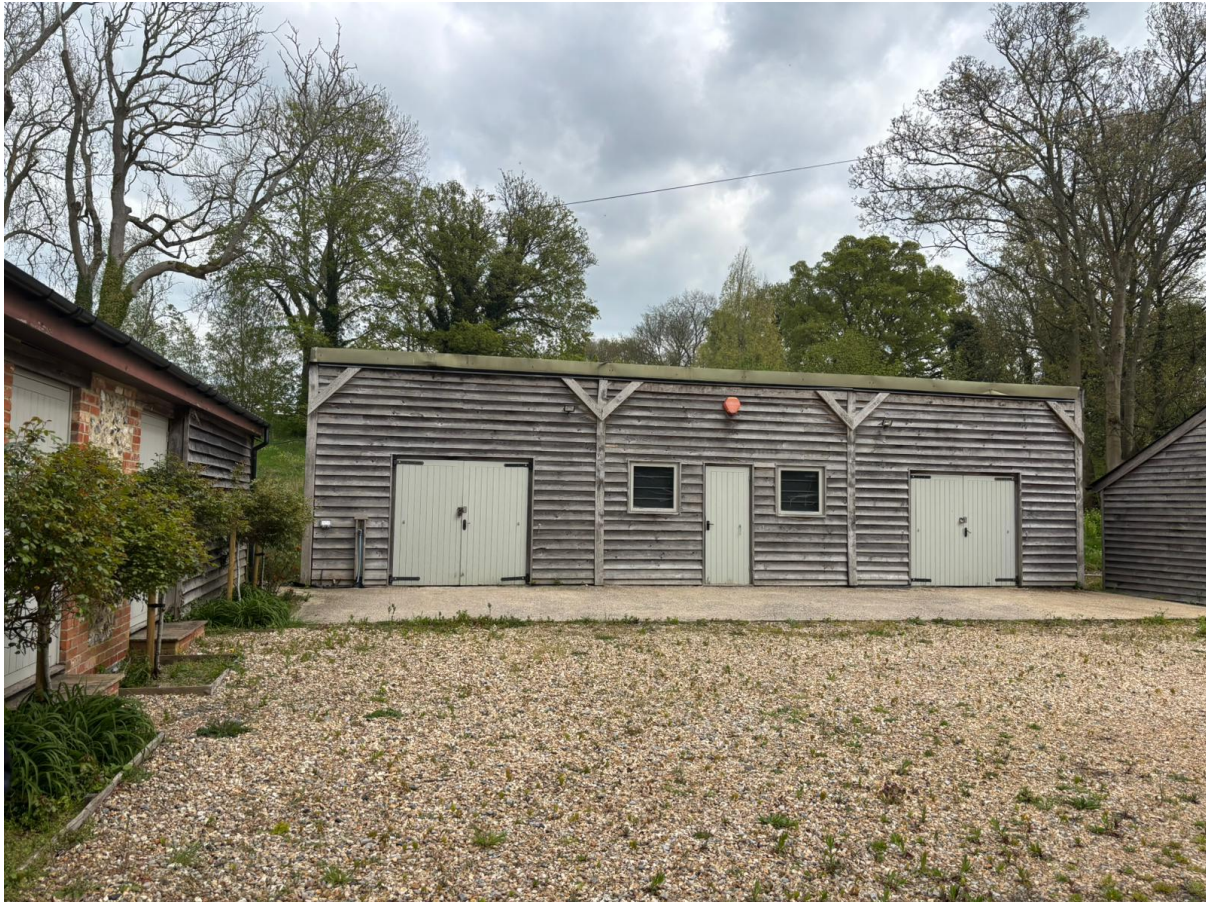
Figure 2 - Existing building to be converted
