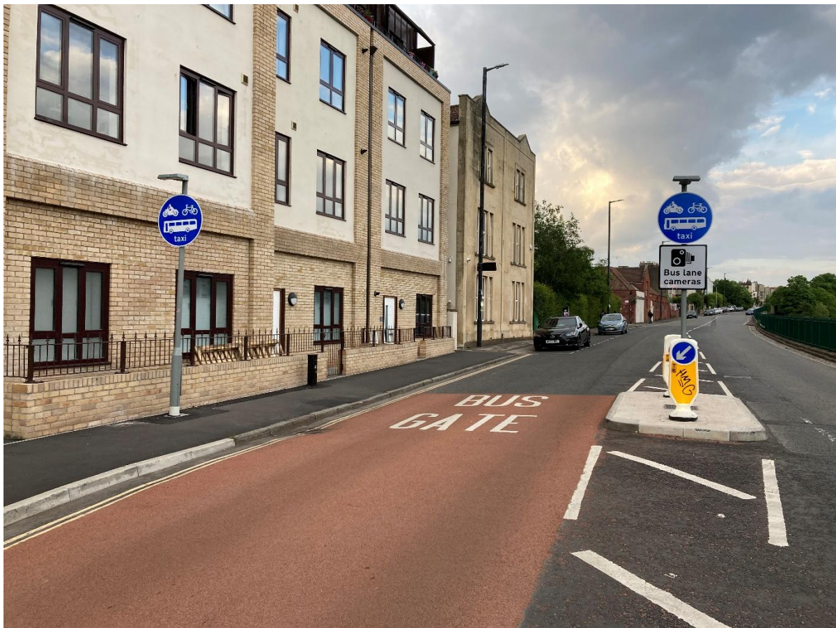
Figure 11 - Example bus gate (Cumberland Road, Bristol)
