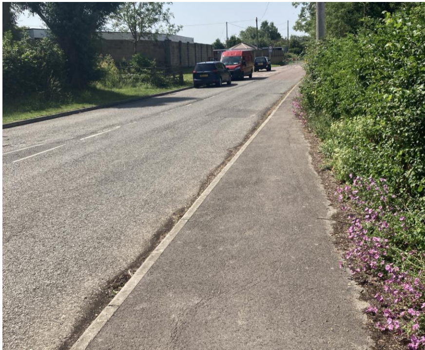
Figure 7: Varying footway widths on Semington Road
