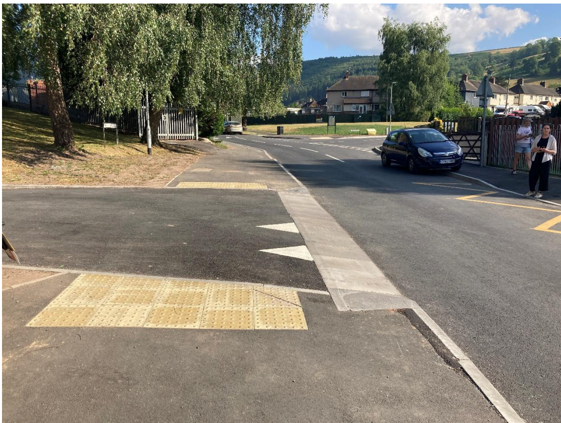
Figure 10 - Example raised side road treatment and footway widening (Llangollen, North Wales)
