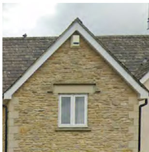
Gables, stone quoins, and window lintel and sill
