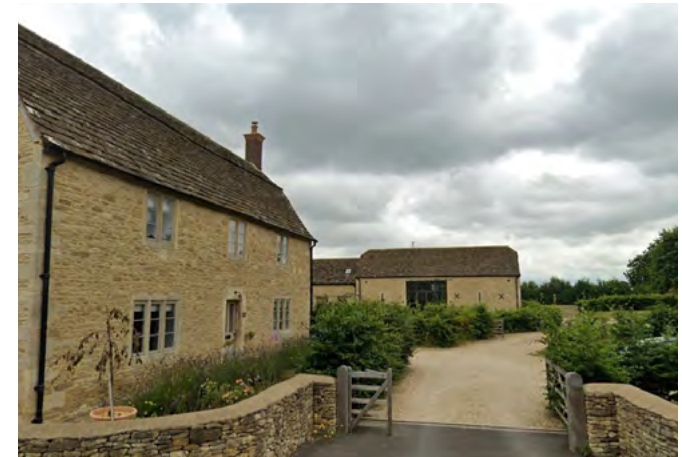
Arms Farm, converted stone farm building
