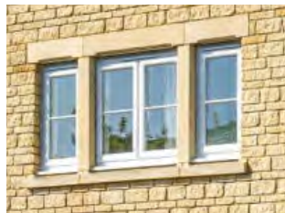
Stone lintel and sill
