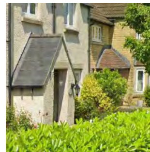
Entrance porches and front gable
