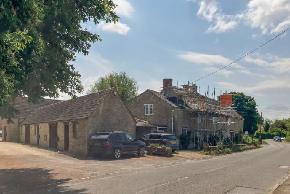
Plate 1. View looking southwest from the western edge of Sutton Benger conservation area
