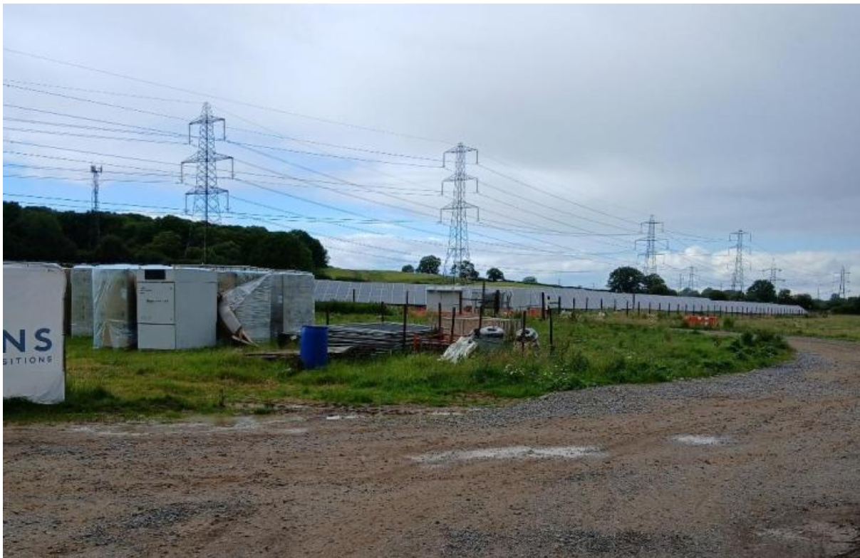
Figure 1: Image taken from site visit in June 2026 from Westlands Lane.
