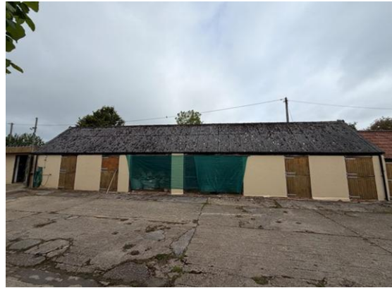
Figure 4: photo of south elevation (LPC)
