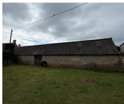
Figure 2: photo of north elevation (LPC)
