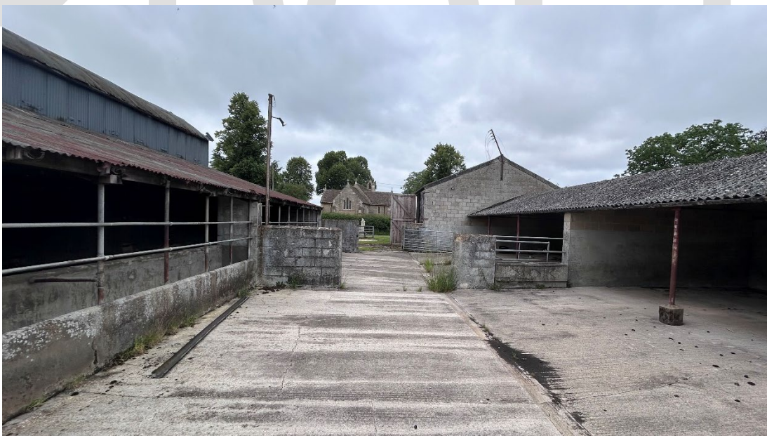
Figure 2 – Application Building (Eastern Range & Byre/Stable Block)
