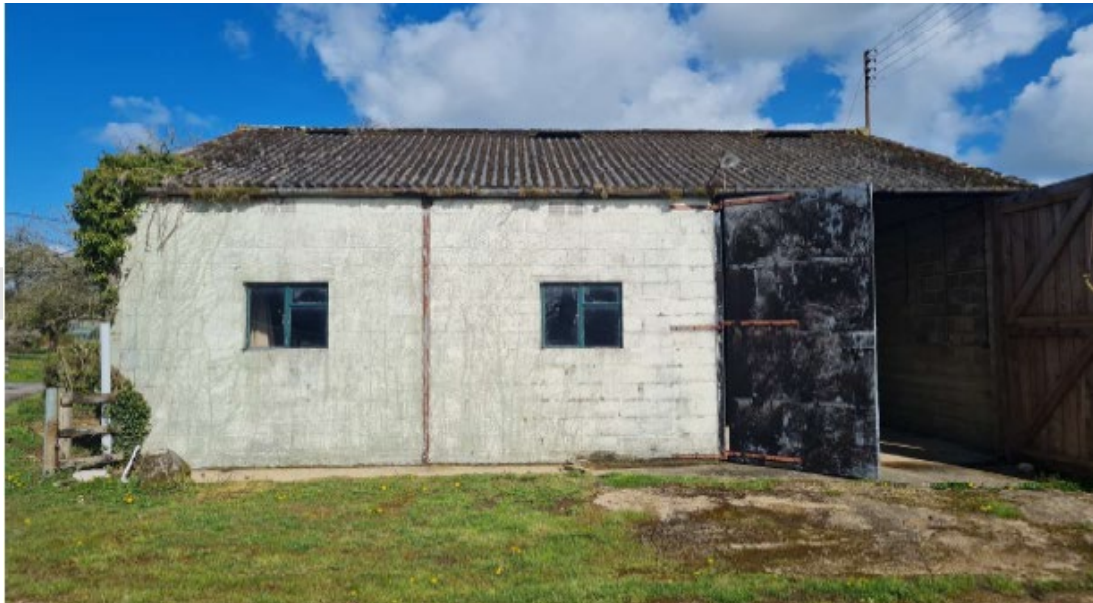
Figure 1 – Application Building (Western Range)
