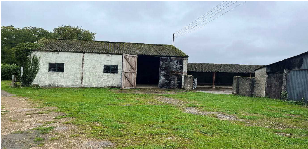
View of barn looking north at southern elevation RWP
