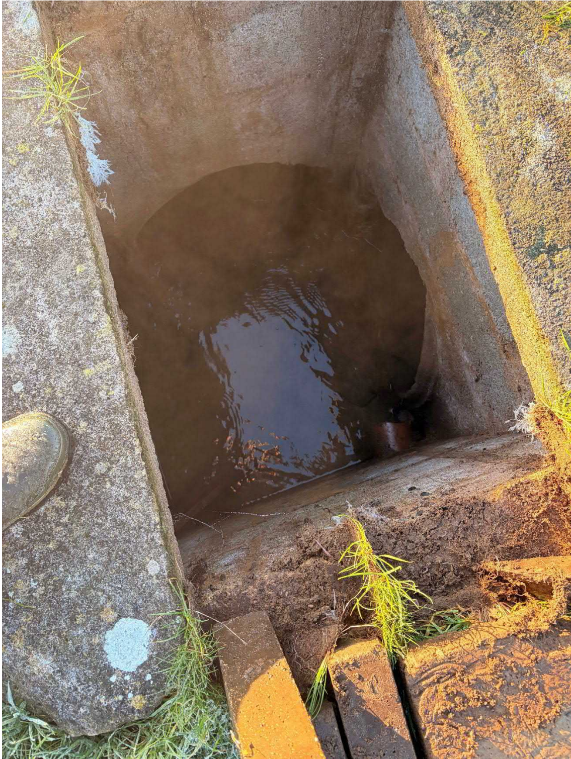
View of the existing manhole located to the northeast corner of the field
