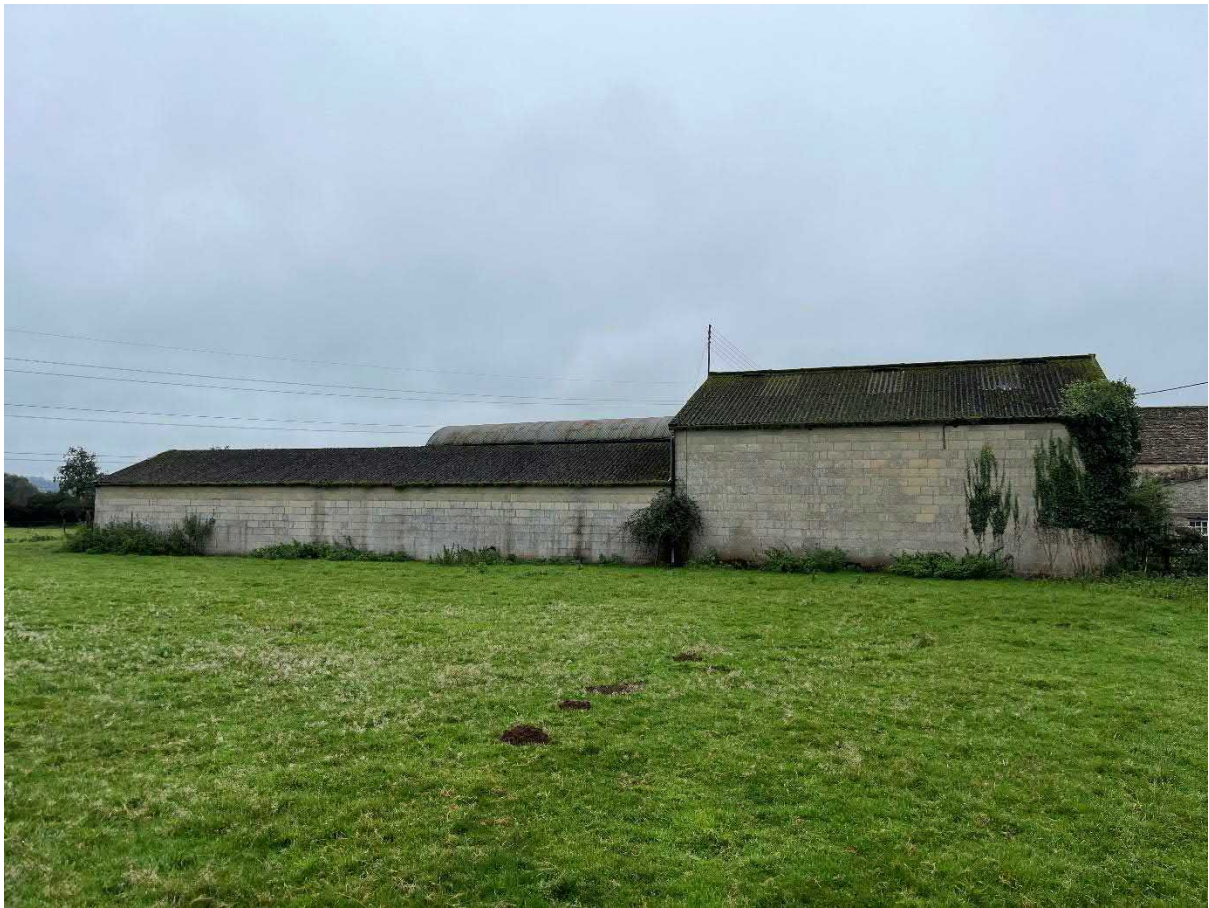
View of Barn northern elevation noting RWPS which drain to eastern corner field drainage system
