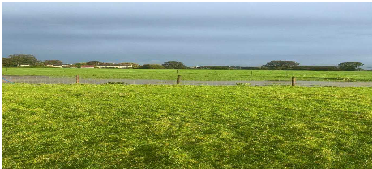
Surface water flowing to the North along field boundary away from the Barn
