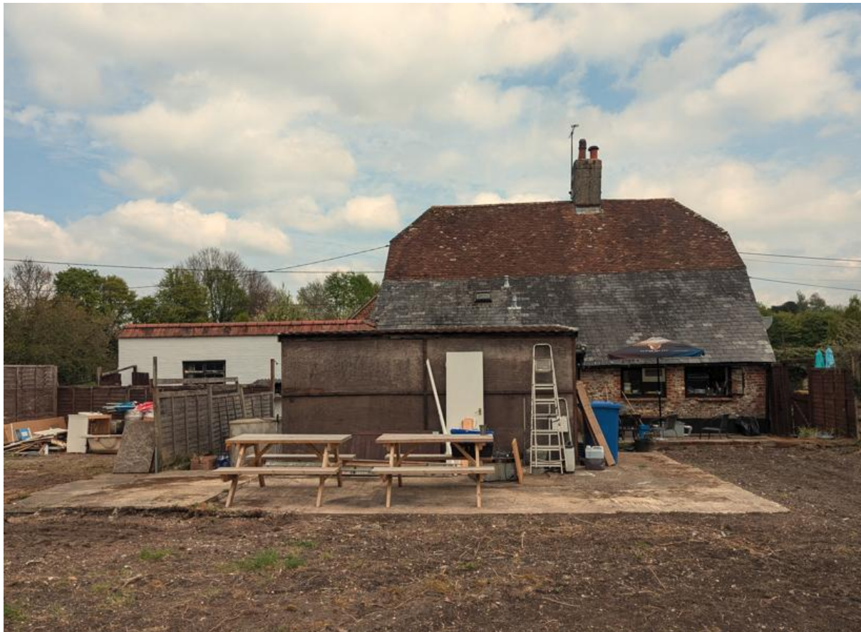
Figure 9 - The site prior to development
