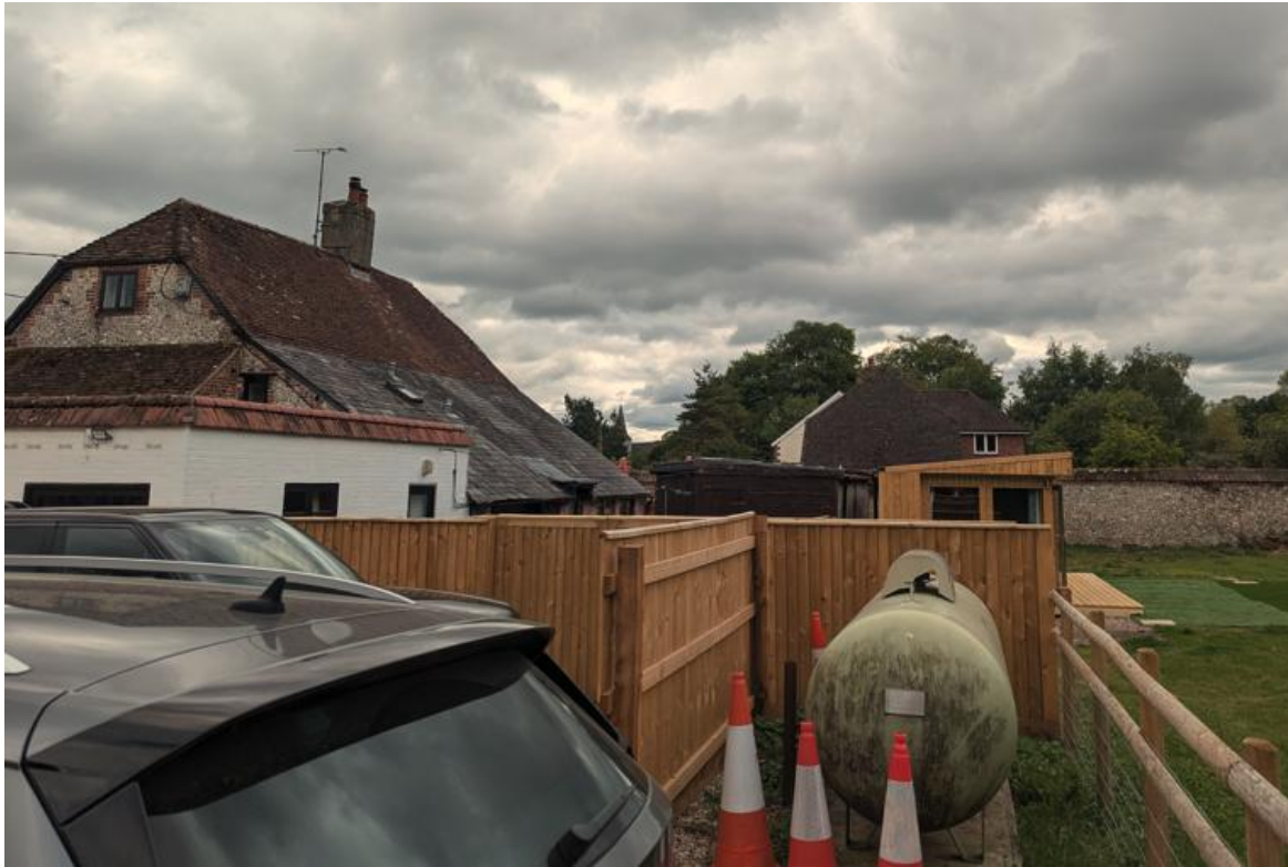
Figure 7 - As built from North
