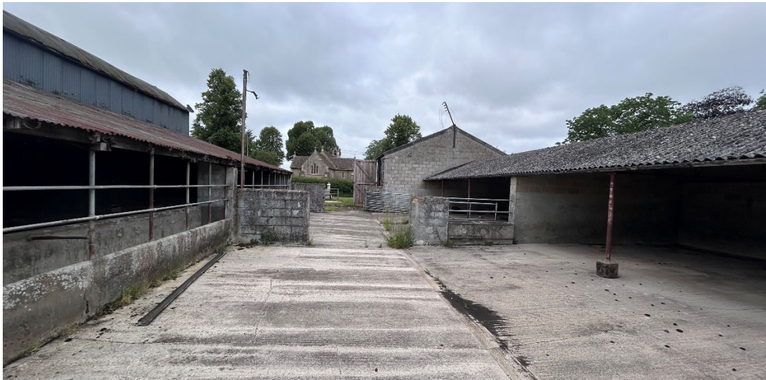
Figure 1 – The application site
